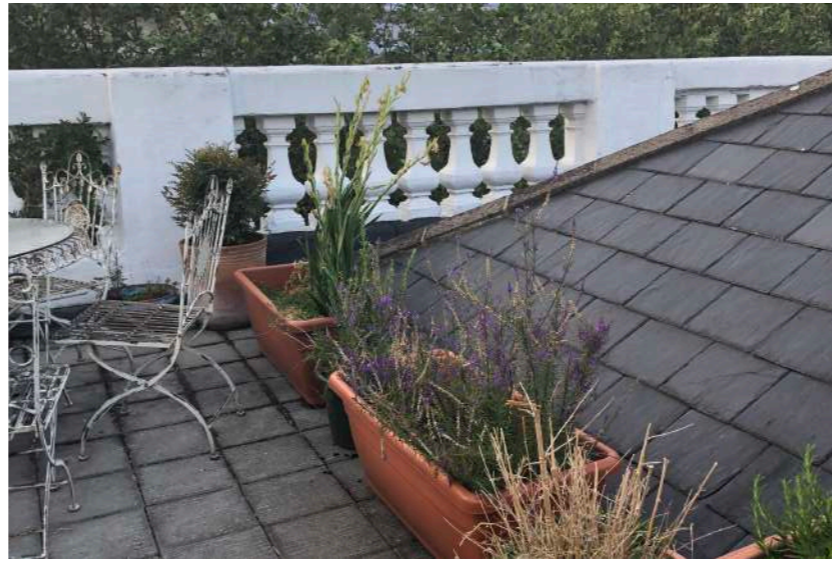
Existing balustrading facing Great Russell Street
