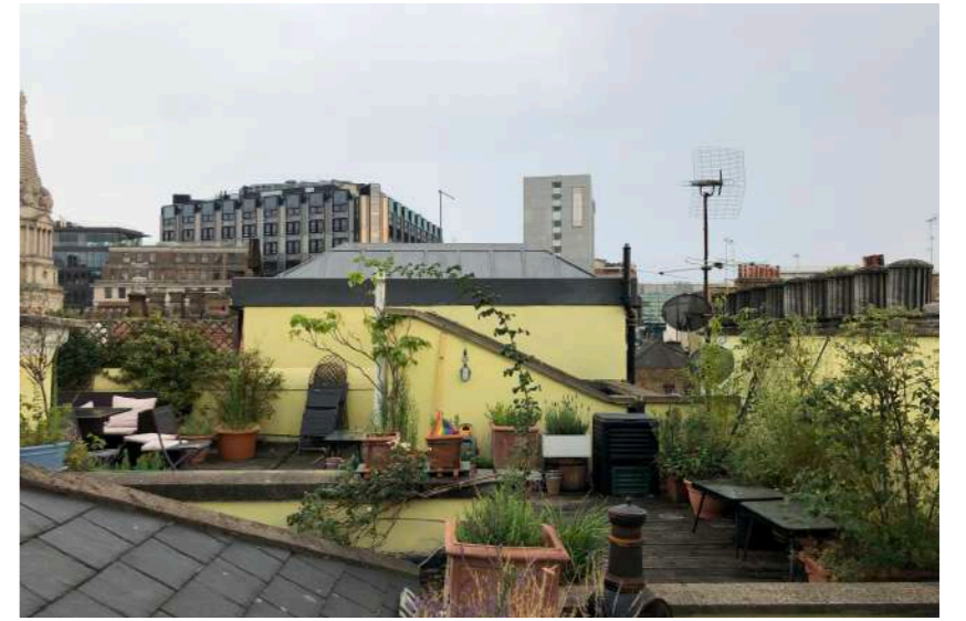
Existing structures and finishes at Nos. 34 & 33 - painted render
