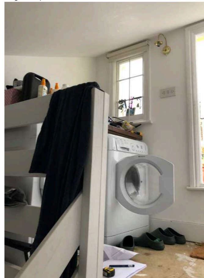
Fig. 3. Photo showing interior of existing roof extension
