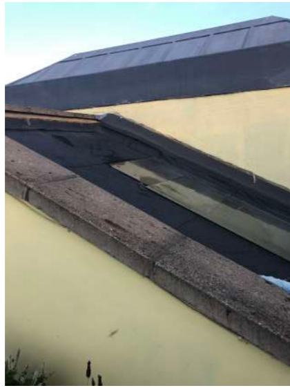
Existing finishes to roof structures @ Nos. 34 & 33
