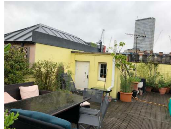
Fig. 4. Photo of existing roof structure adjacent to existing roof structure at No. 33
