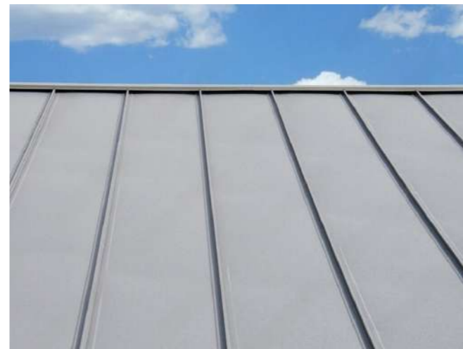
Fig. 6. Sample finish to standing seam zinc roof
