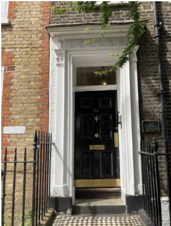
Main Entrance Door
