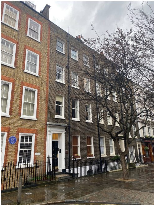
Fig.03: Existing building: 22 Great James St, highlighting the entrance.
