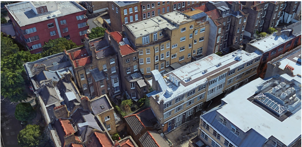
Fig.05: Existing building: 22 Great James St, highlighting the rear closet storeys
