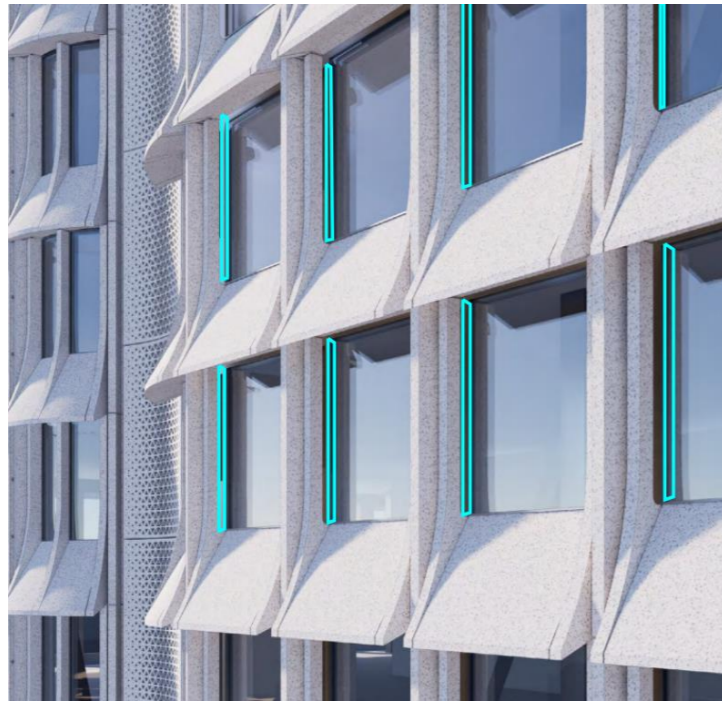
Figure 5: Example of curtain wall façade panels showing solid elements and shadow gaps around glazing for natural ventilation
