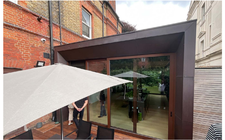
Rear of side extension
