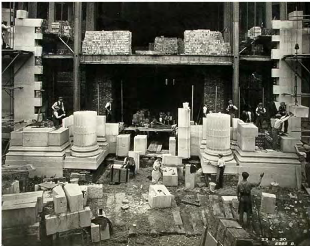
Plate 16: Early 20th century hall under construction
