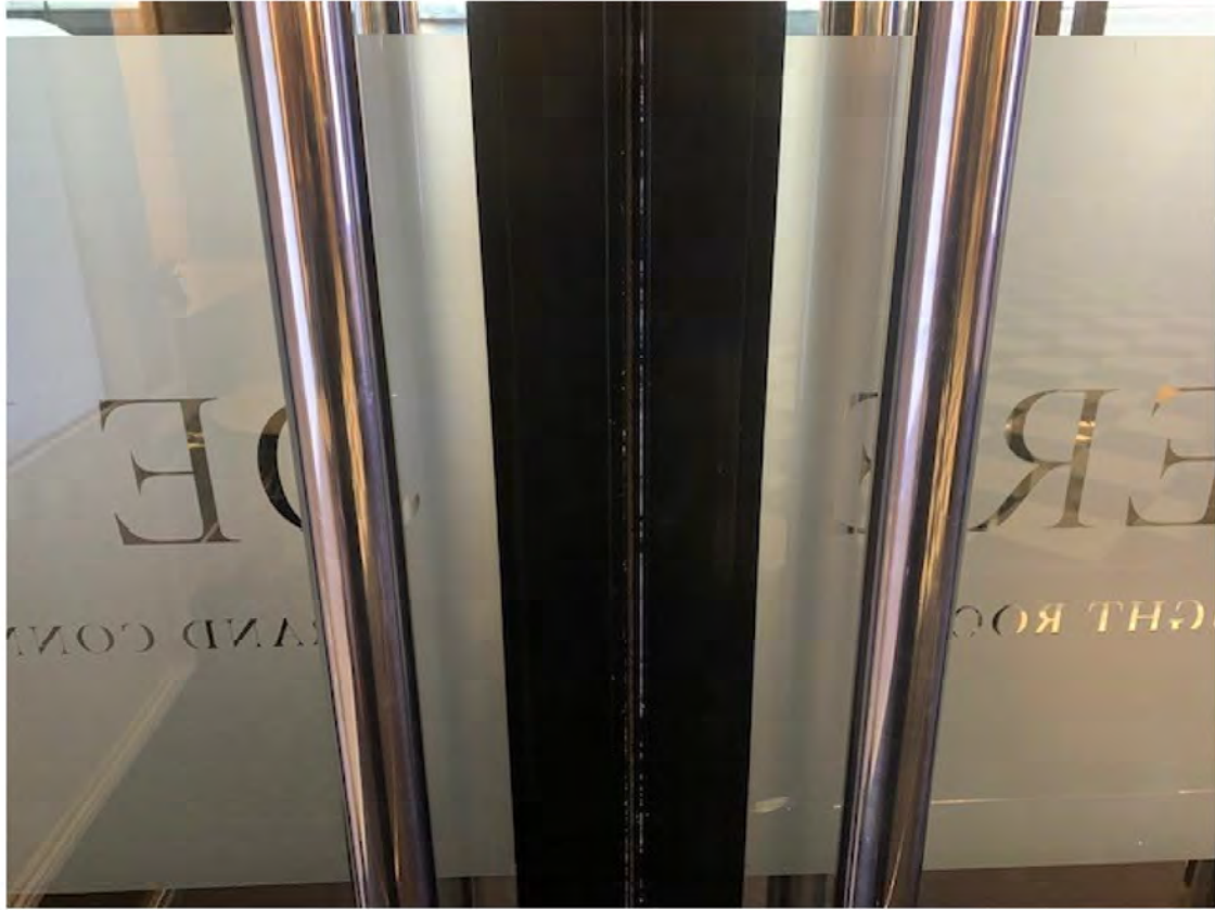
Plate 1: Detail of central junction and handrails
