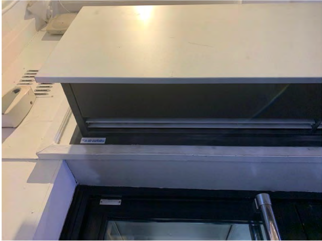
Plate 3: Junction between door and overhead heater
