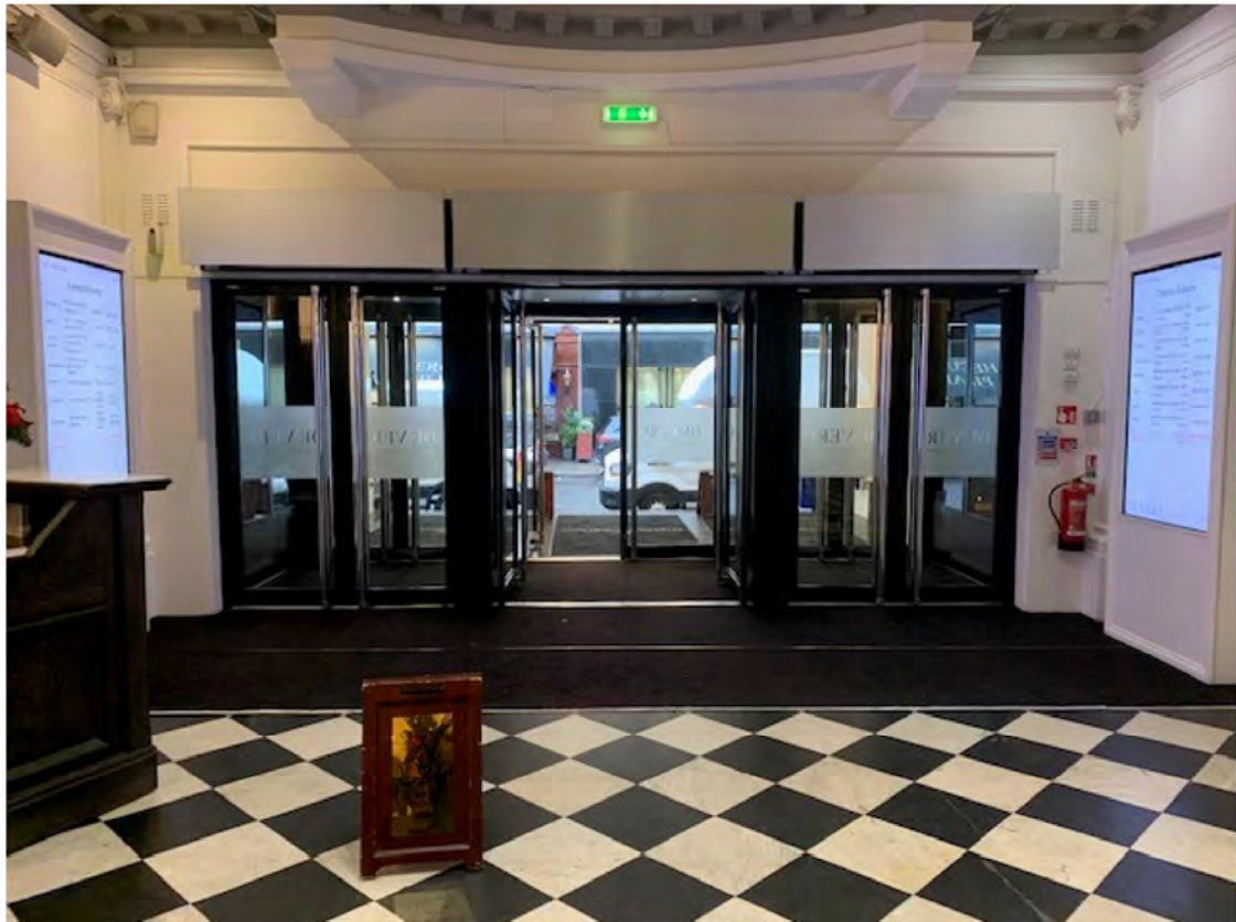
Plate 4: Elevation of doors from interior
