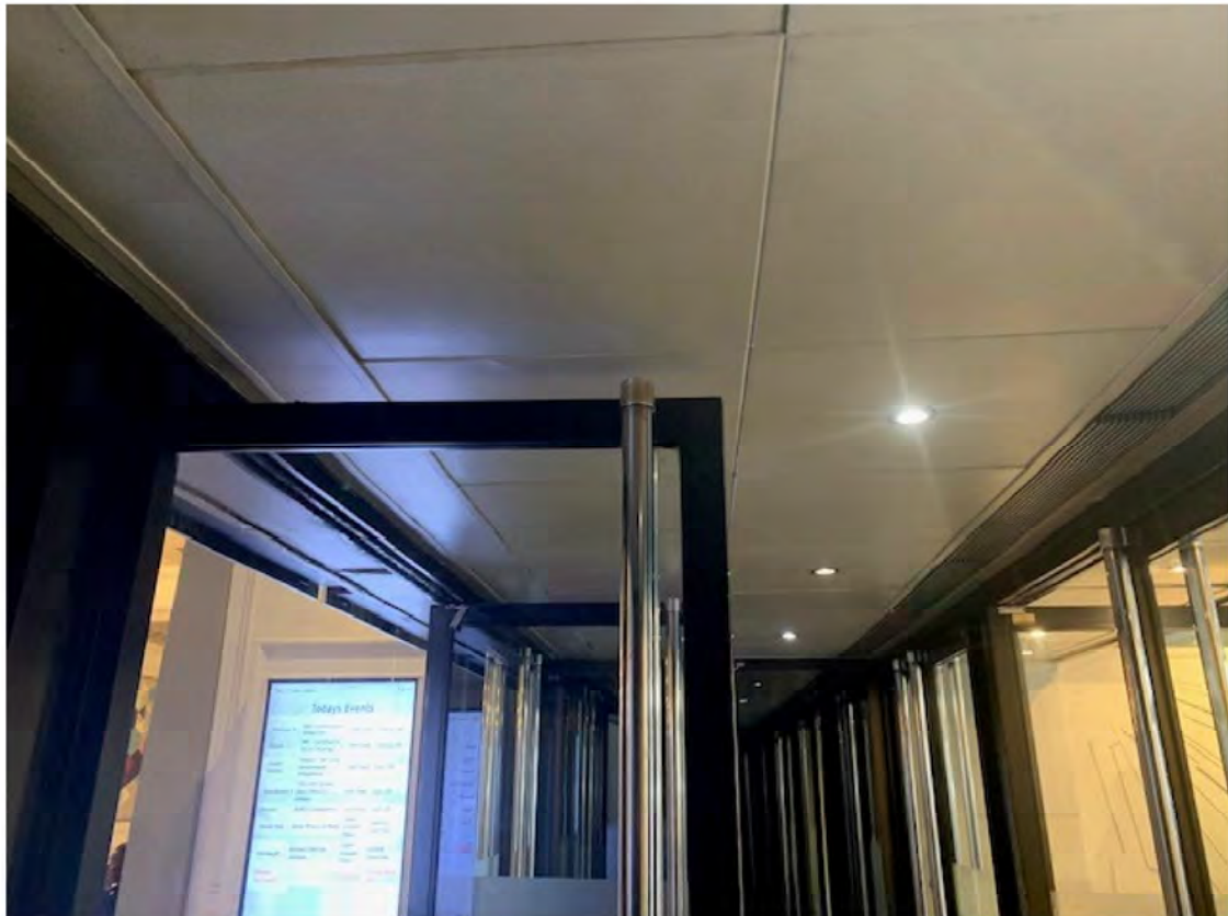
Plate 6: Ceiling within lobby
