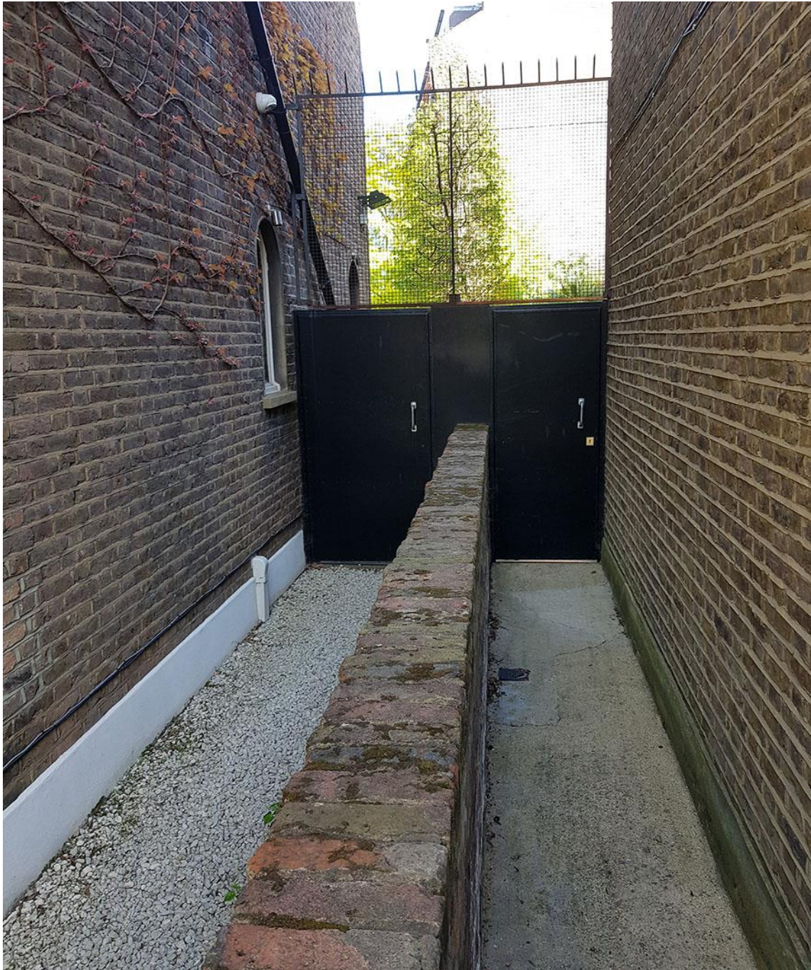
Image 3. Showing the existing gate along the flank elevation
