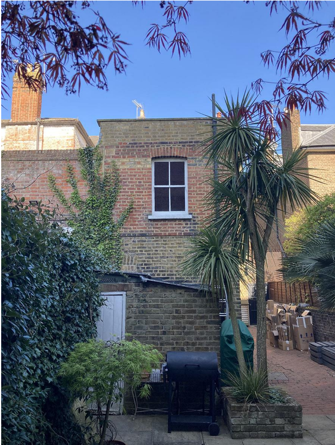
Image 4. rear elevation, looking west
