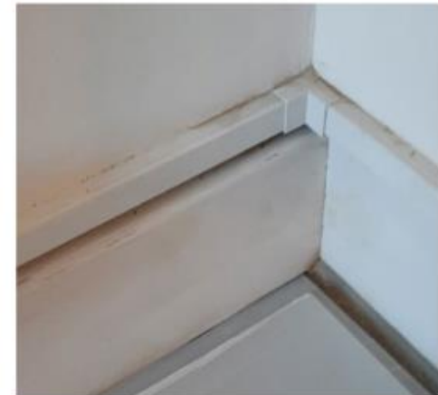
Proposed finished skirting board in pilot flat
