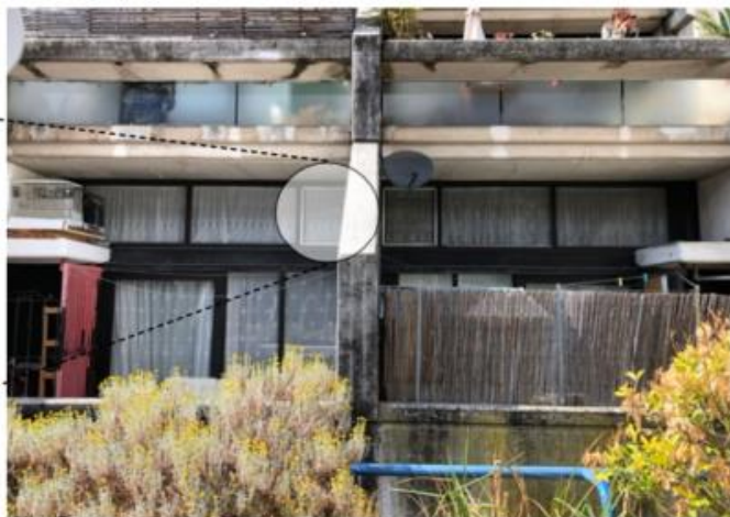
Photo of bottom hung inward opening window as built in 26A pilot flat.
