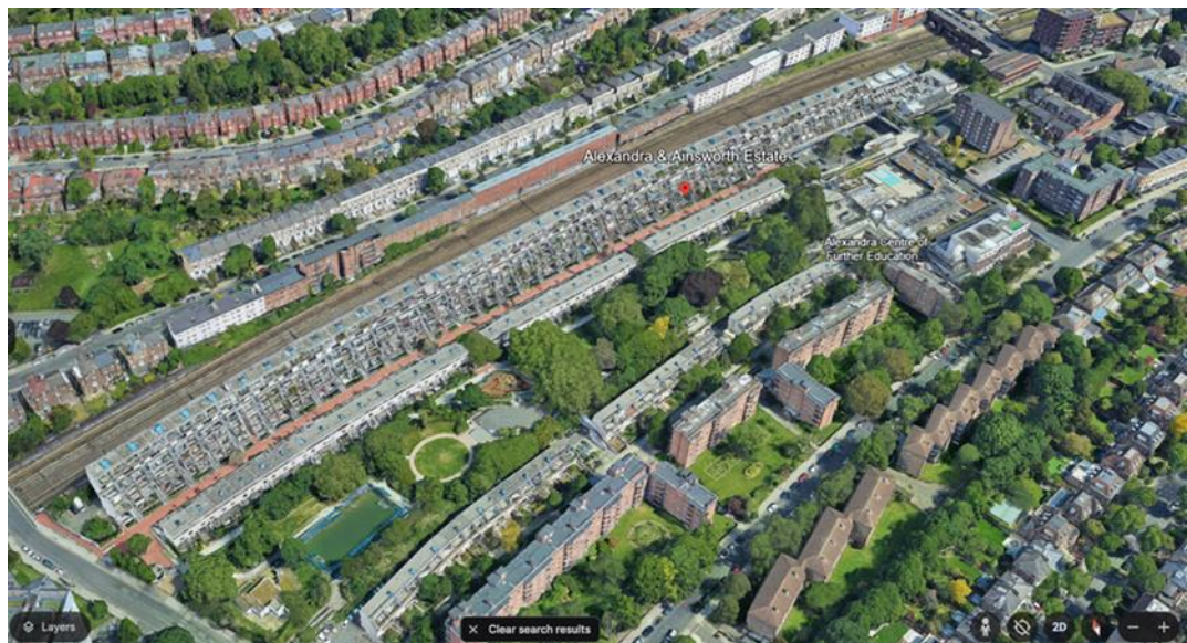
Figure 1 – The existing site
