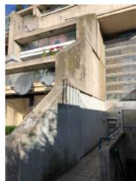
Figure 4.2 - Rear of block A showing the heated party wall from the coils and the unheated wall
