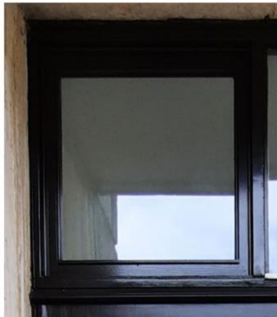
Photo of bottom hung inward opening window as built in 26A pilot flat.
