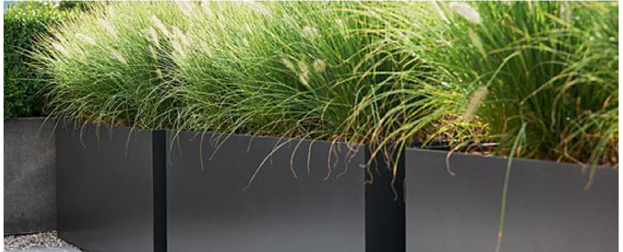
Metal planter on green roof
