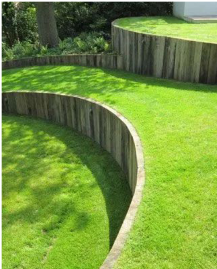
Timber retaining wall
