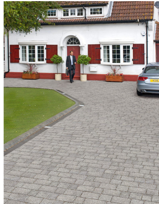
Permeable concrete sets
