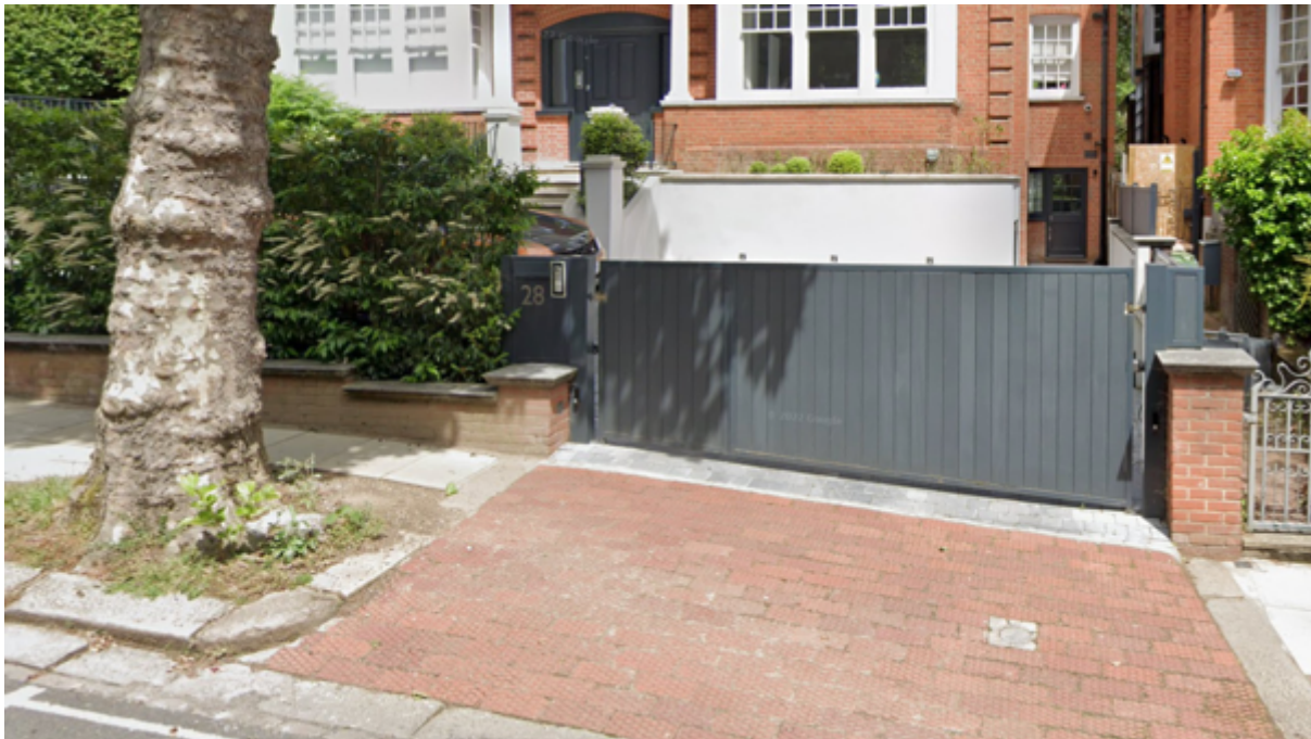
As Built Photograph (28 Ferncroft Avenue)
