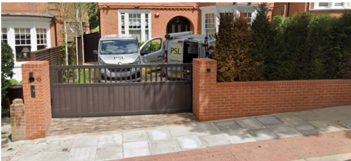
As Built Photograph (10 Ferncroft Avenue)
