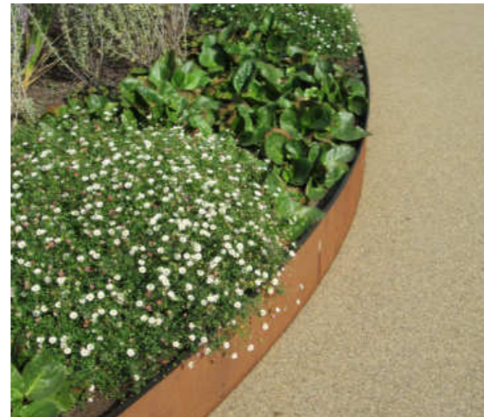
Raised steel edge
