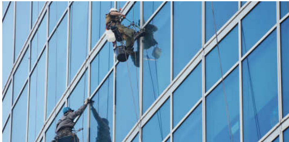
Rope access façade maintenance example
