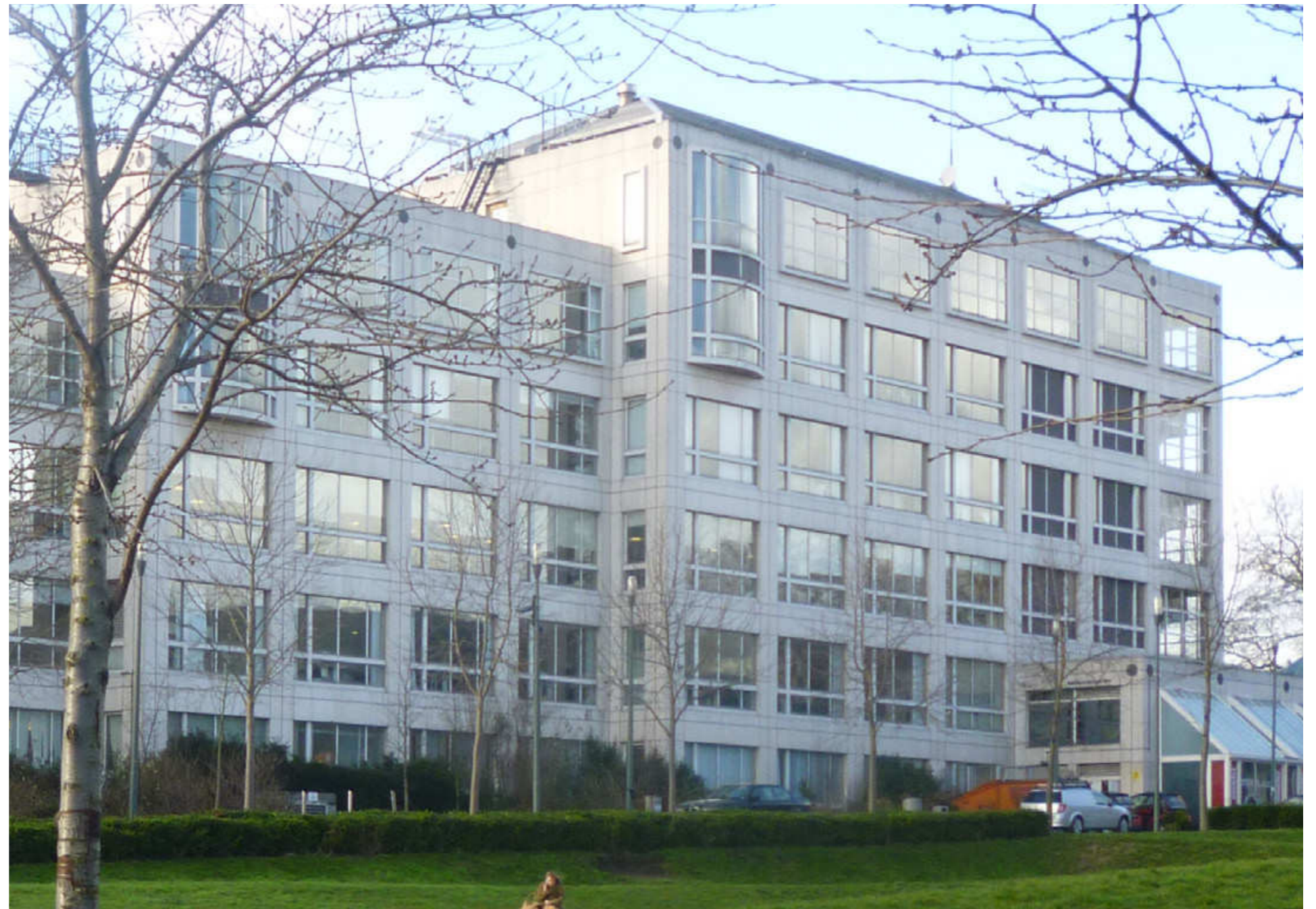
Former Office Building - Pre-Demolition
