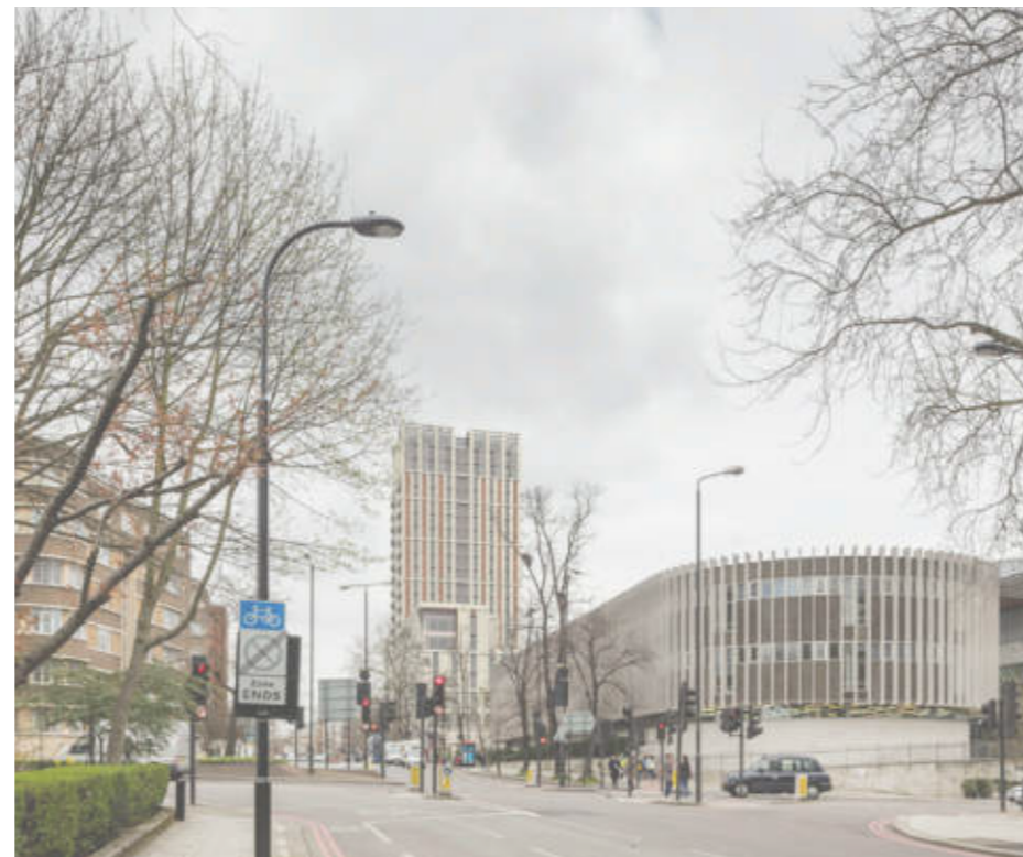
View looking North along Avenue Road - Extant Permission
