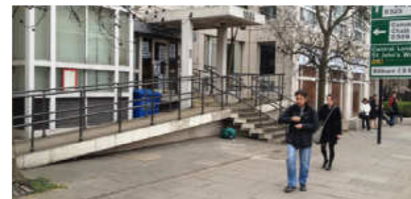
Former Office Building Entrance - Pre-Demolition
