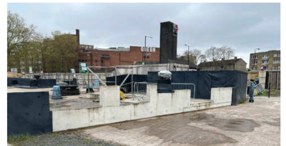
Consented Ground Slab - Site Condition
