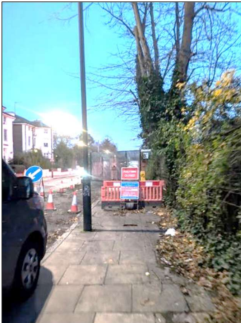
Photograph 4D: Closed footway along Adelaide Road
