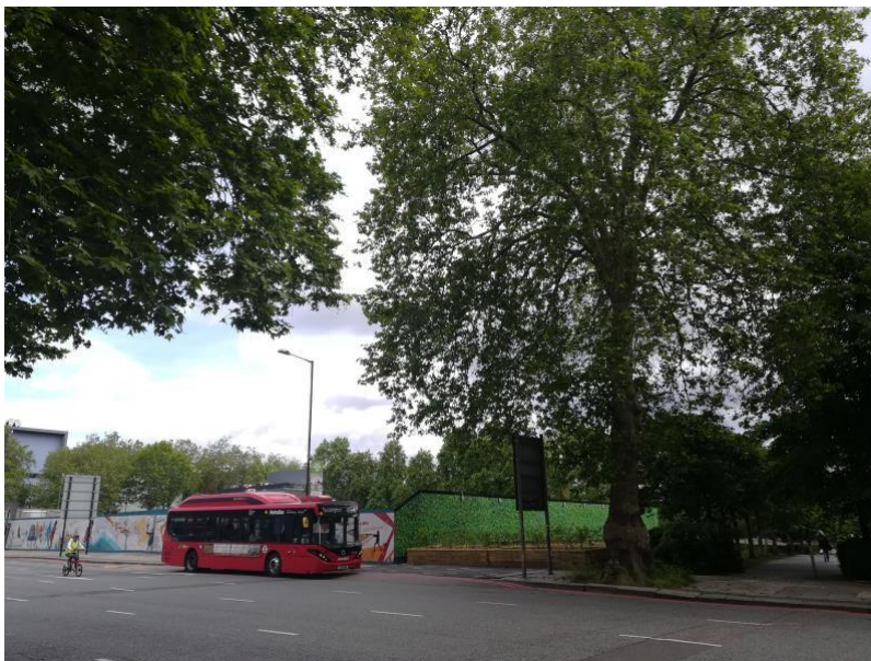
Figure 9: The temporary crossover that has been installed adjacent to T1 (to the right of the bus)
