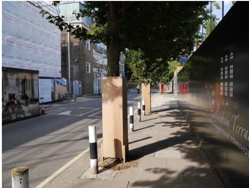
Figure 10: Example of plyboard box stem protection that can be used on street trees.
