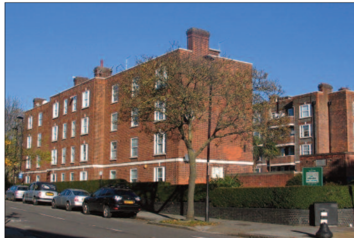
▲ Torriano Estate, was built in the 1930's and designed by A. J. Thomas who built Kennistoun House (on Camden's Local List) and Camden Town Hall (Grade II listed).
