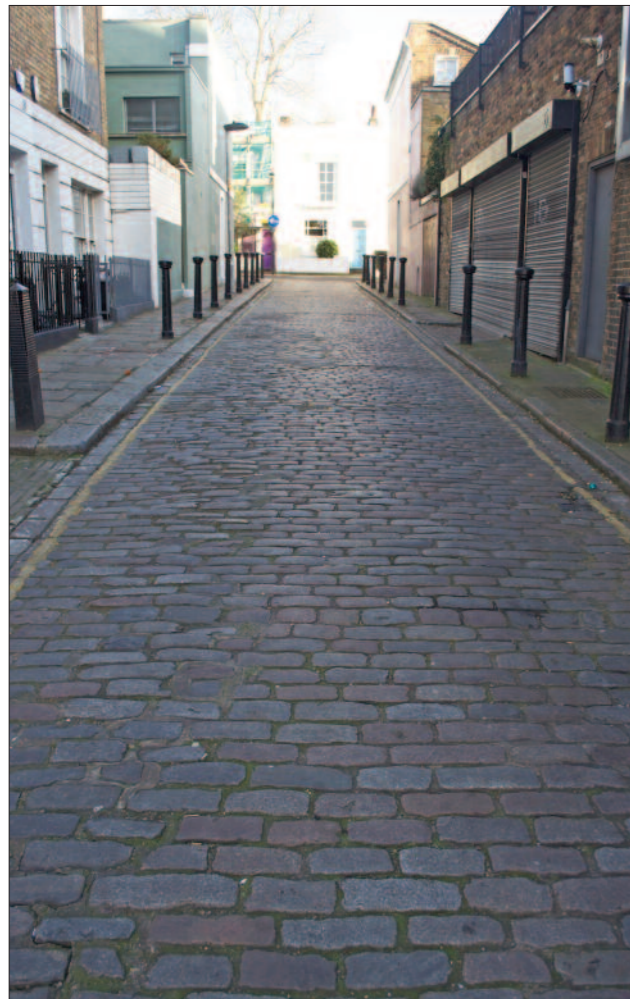
▲ Leverton Place is a rare example of a virtually intact and continuous granite setted carriage way. Continuity is broken only by some patching and a break where it intersects with Leverton Street. The high quality of setts, gutters and kerbs creates a consistency of setting for the variety of building types in this lane.
