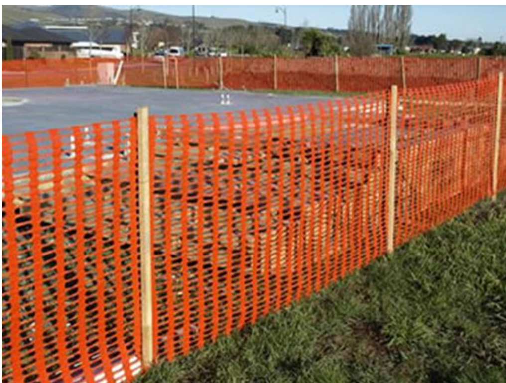
Figure 8: Example of hi-visibility barrier tape fencing secured with timber stakes (Image supplied by Honesty & Faith Hardware Products Co. Ltd).
