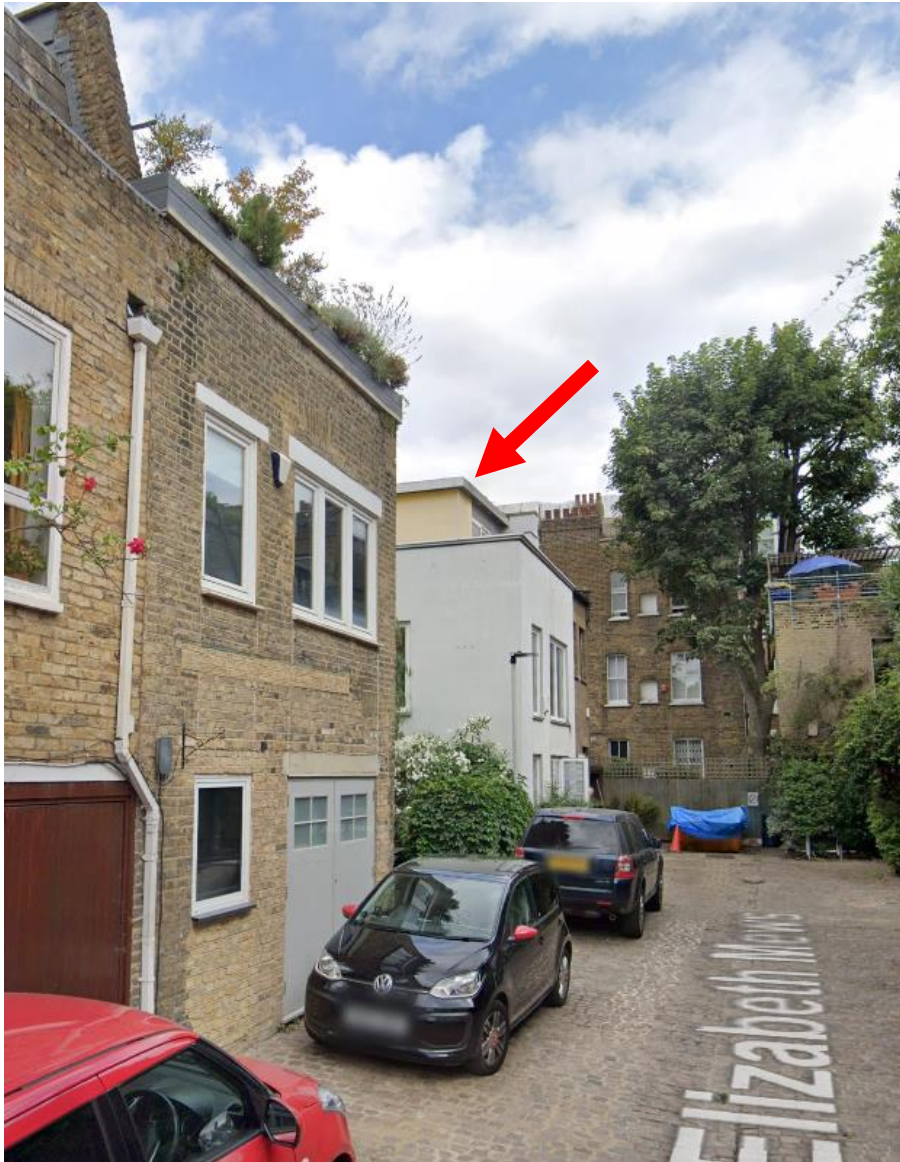
Fig 3. Subject site (left) and neighbouring no.11a with roof extension (red arrow)
