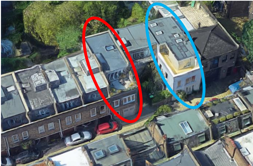
Fig 1. Aerial view of 11 Elizabeth Mews (red) and neighbouring no.11a (blue) with extension.
