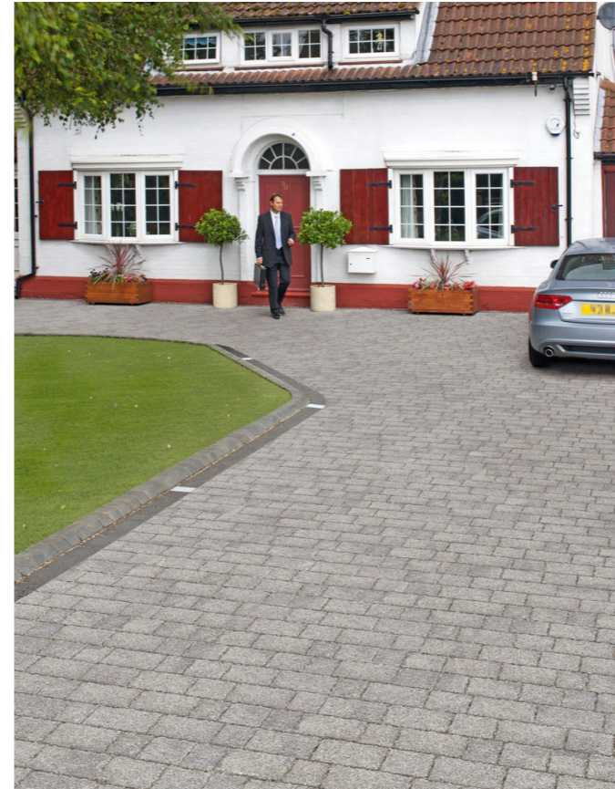
Permeable concrete sets
