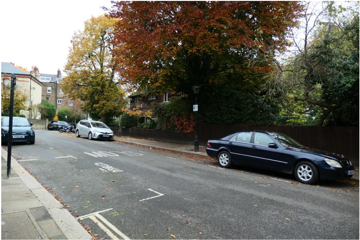
Photo 12: An oblique view of the façade, from Pilgrim's Lane.
