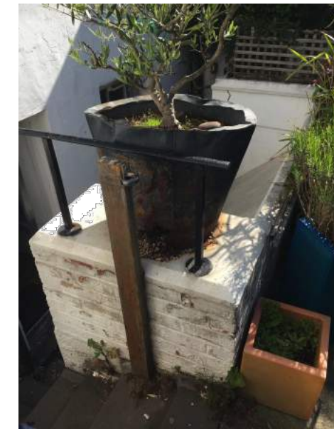
D VIEW LOOKING DOWN TO THE BASEMENT STEPS + RETAINING WALL
