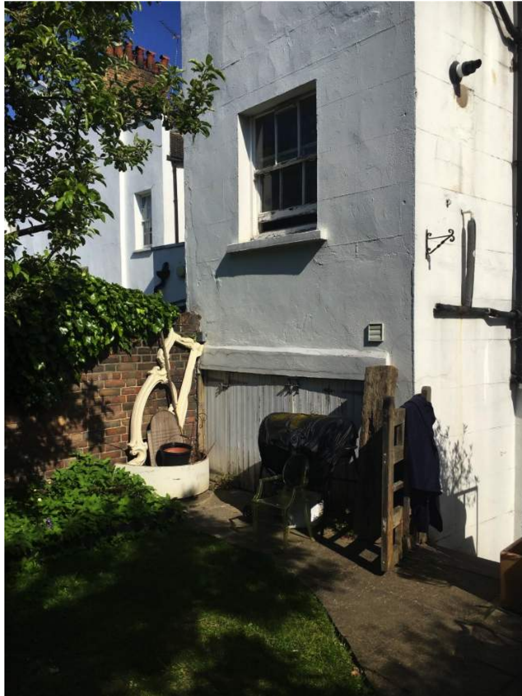
A VIEW FROM THE REAR GARDEN LOOKING TOWARDS THE PROPOSED STAIRCASE TO THE REAR OF THE HOUSE
