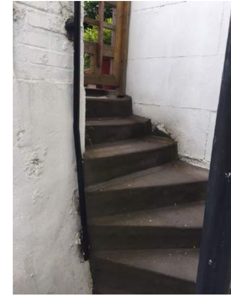
C VIEW LOOKING UP FROM THE BASEMENT STEPS
