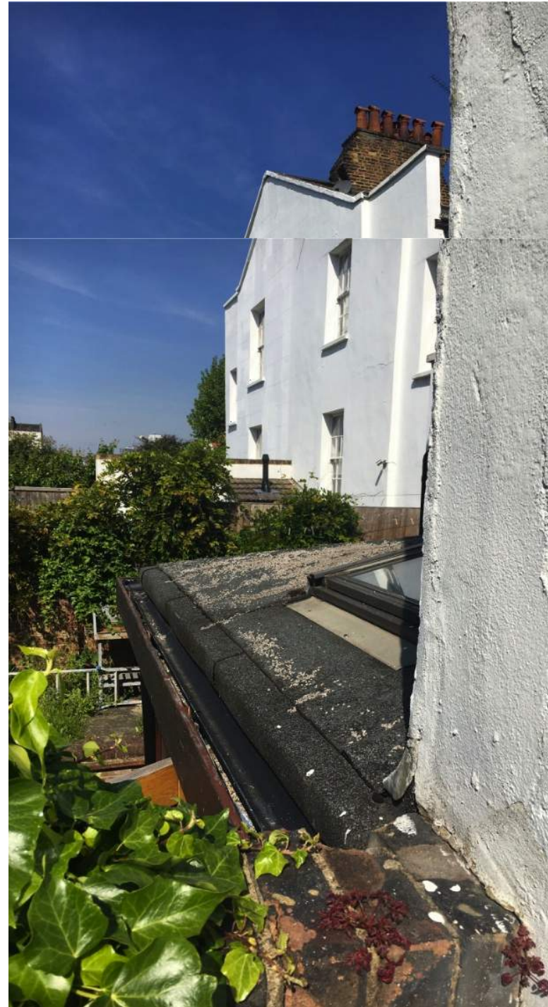
B VIEW FROM THE GARDEN WALL TO NUMBER 24 LOOKING AT THEIR REAR EXTENSION
