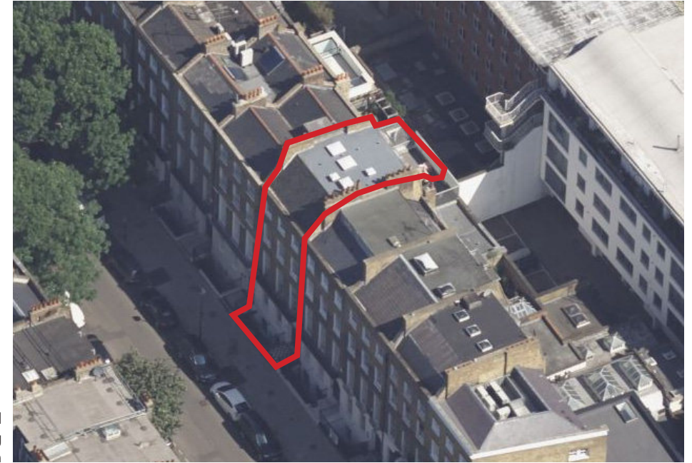
View 01 Aerial view looking North
