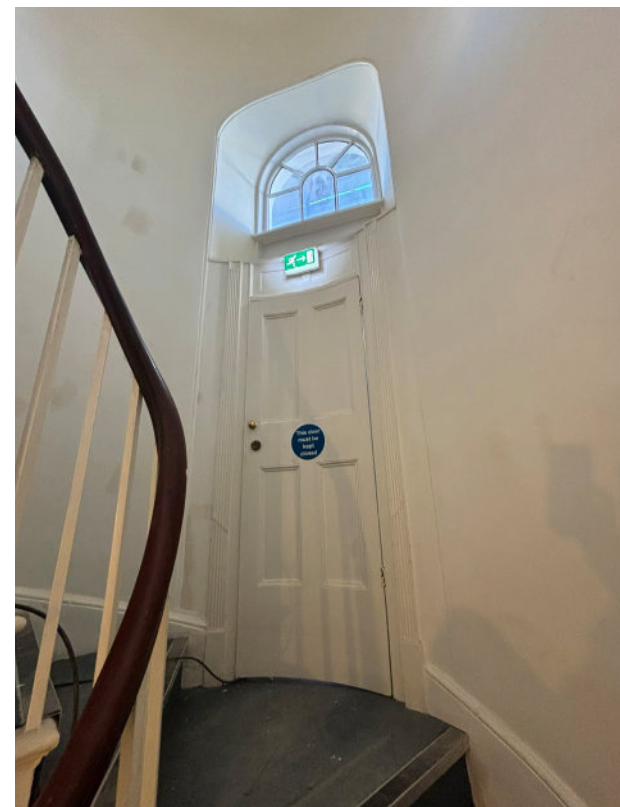
3. First to Second Floor Landing. View of the door to the existing closet wing.
