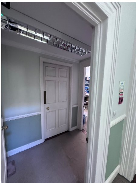
Figure 12: A view into the subdivided front room from the 1st floor landing showing the modern suspended ceiling to the lobby area.
