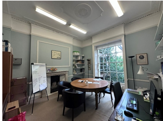
Figures 13 & 14: Internal views of the front and rear rooms at ground floor level showing cornicing, decorative plasterwork, window shutters and roundel detailed fireplaces.
