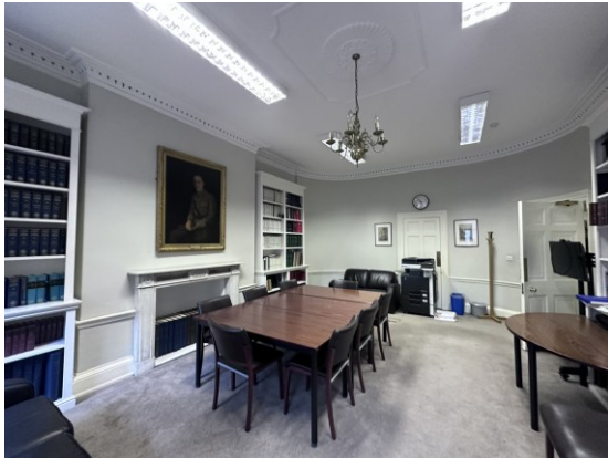
Figures 13 & 14: Internal views of the front and rear rooms at ground floor level showing cornicing, decorative plasterwork, window shutters and roundel detailed fireplaces.
