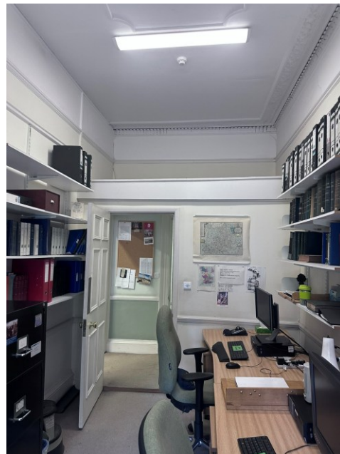
Figures 15 & 16: The narrow space formed by modern partitions to the front space at 2 nd floor level and the very obvious suspended ceiling to the lobby formed within the front 1 st floor room.
