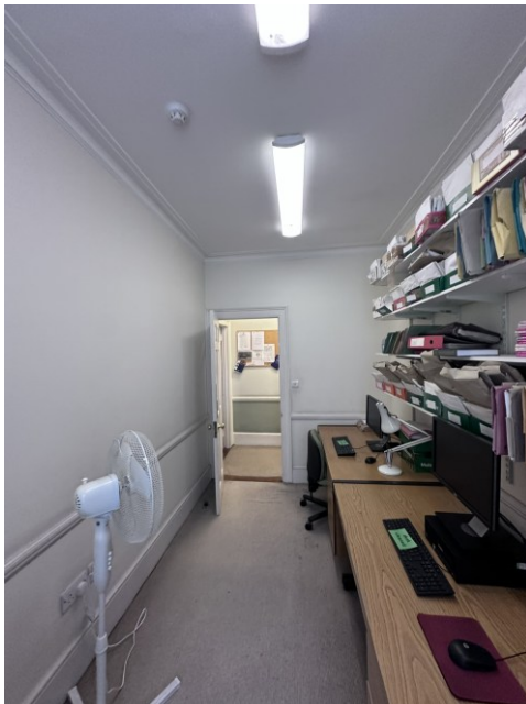
Figures 15 & 16: The narrow space formed by modern partitions to the front space at 2 nd floor level and the very obvious suspended ceiling to the lobby formed within the front 1 st floor room.
