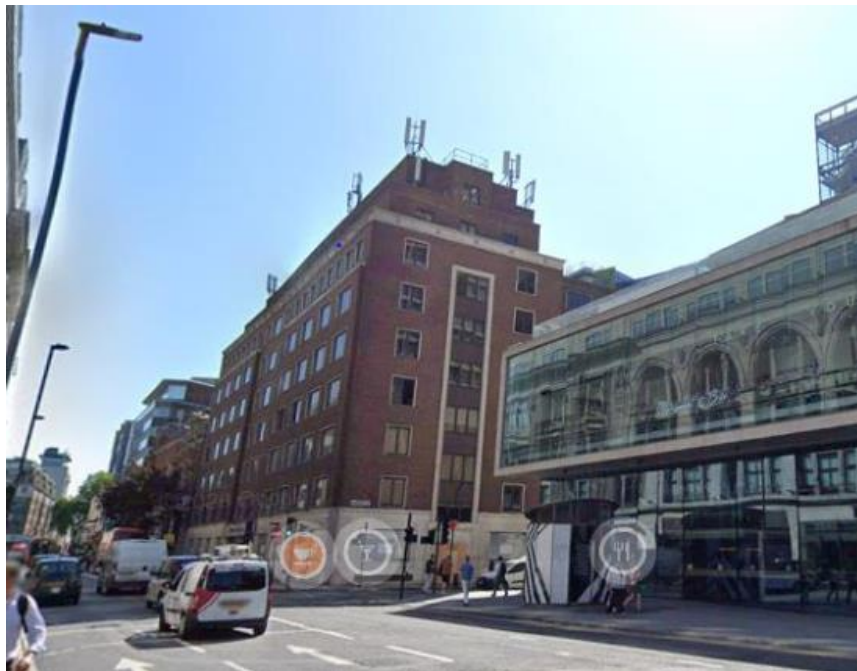
Figure 2 - View of the former Castlewood House from Castle Point from New Oxford Street (west)
