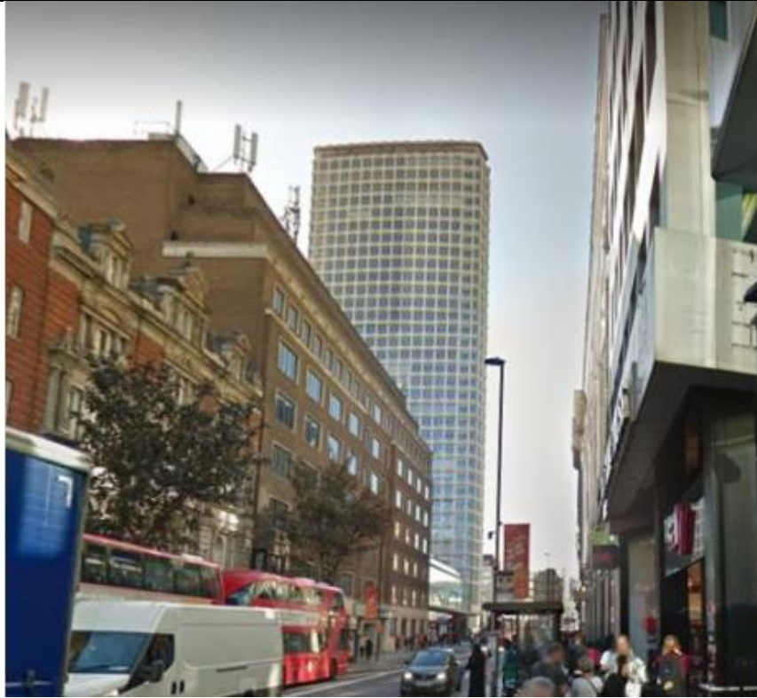
Figure 3 - View of the former Castlewood House from New Oxford Street (east)
