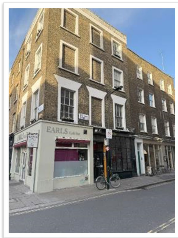
Fig.14: A different arrangement of blind windows in Shelton Street
