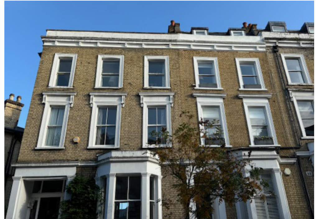
Existing Front Elevation - mansard roof extensions at 40 and 41 Gayton Rd visible
