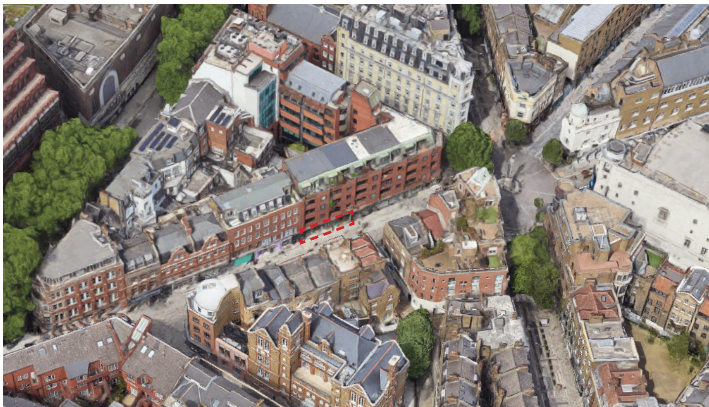
Existing building aerial photo
