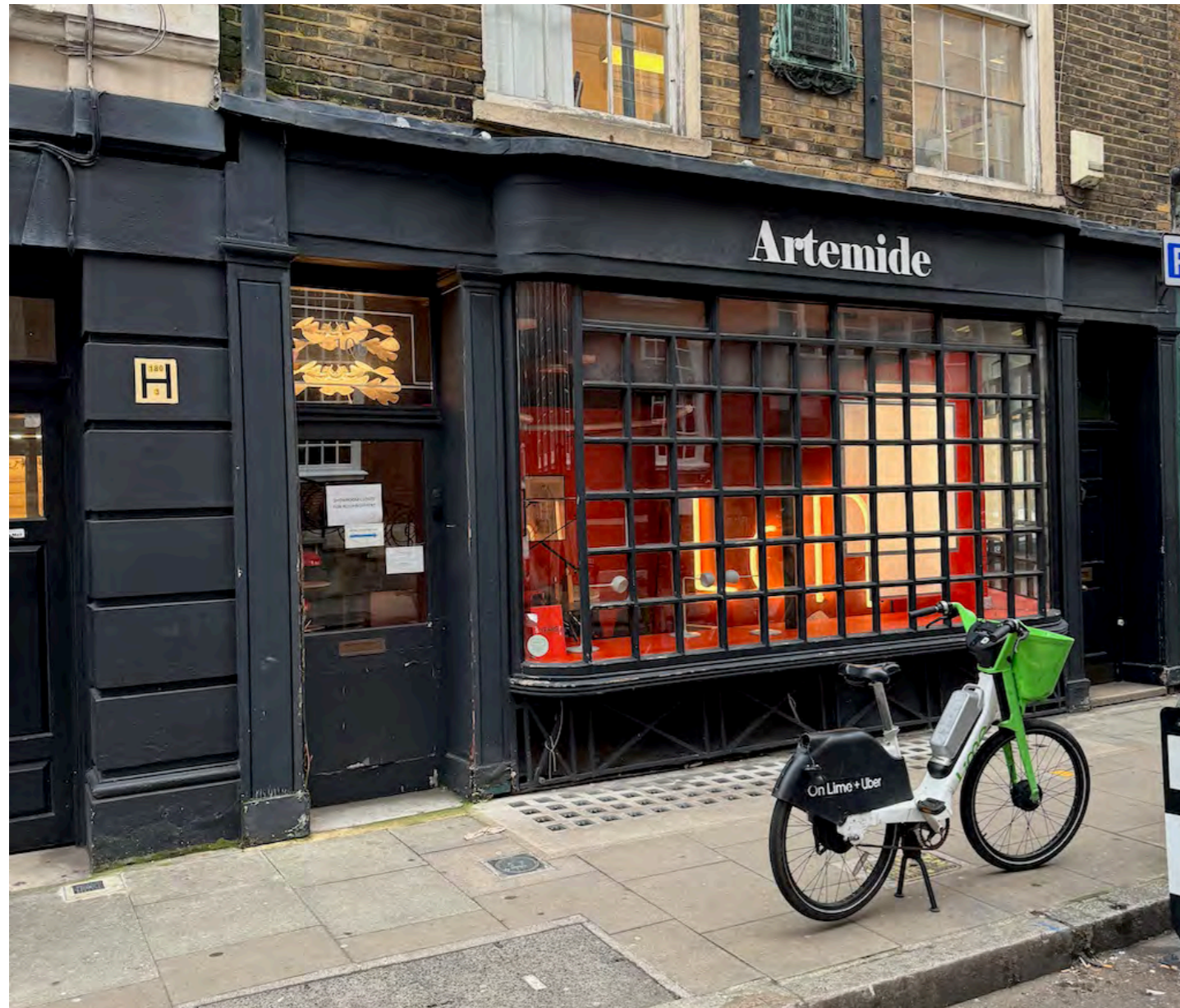
The existing shop front has 2 door entrances and is categorised by a timber projecting window. The ends of the projecting window have a distinct curved glazed frameless window.
