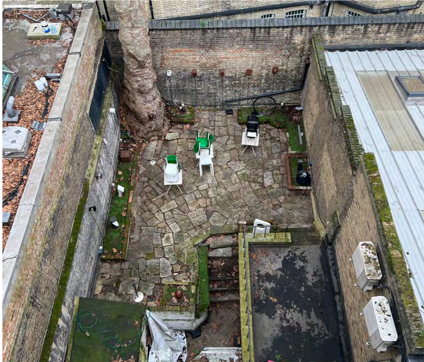
The photograph above illustrates the full rear extensions of the neighbouring properties in relationship to the site at 106 Great Russell Street.
