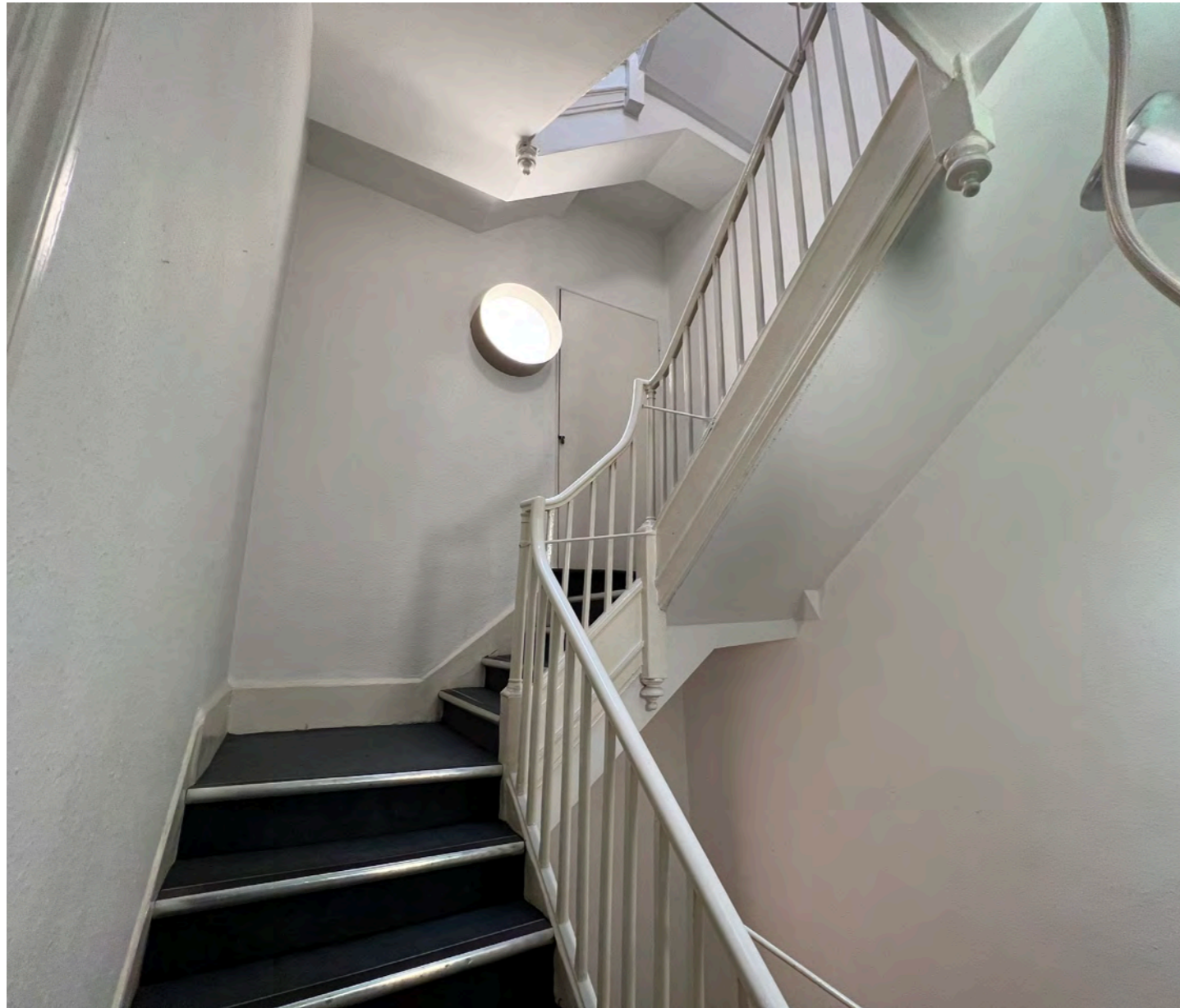
The photograph above illustrates the main staircase.
