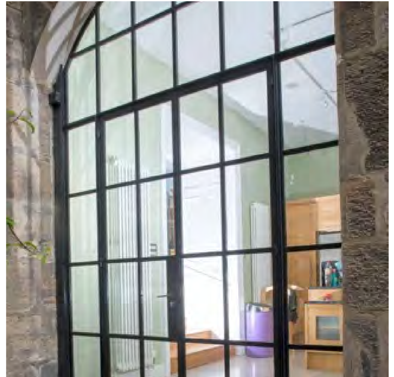
The Crittall glazing above illustrates how well the glazed proportions of this system will compliment the proposed design for new glazing system at lower ground level, whilst maintaining the heritage of the existing property.
