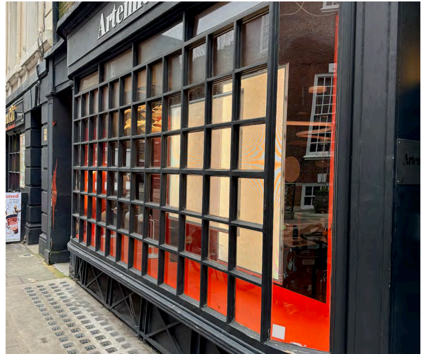
Photograph above of the projecting window with the distinct curved glazed frameless window.
