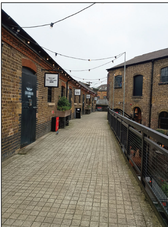
Figure 3: First floor Stables and walkway
