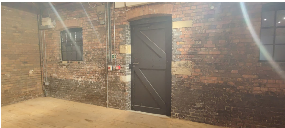
Figure 3: Interior view of one of the seven units
