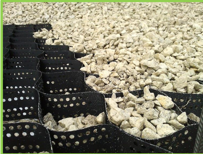
Arboricultural Protection Method 2 – Temporary Ground Protection
