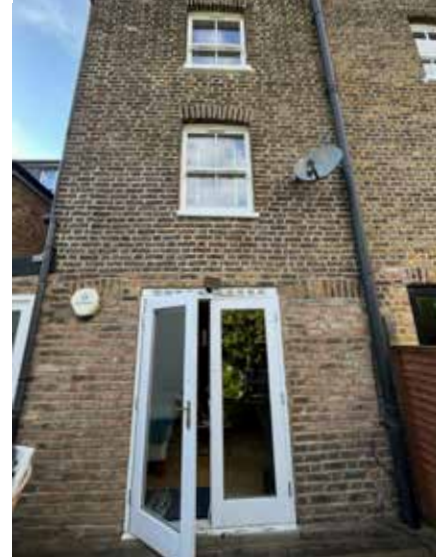
Existing rear elevation. Picture taken: May 2024
