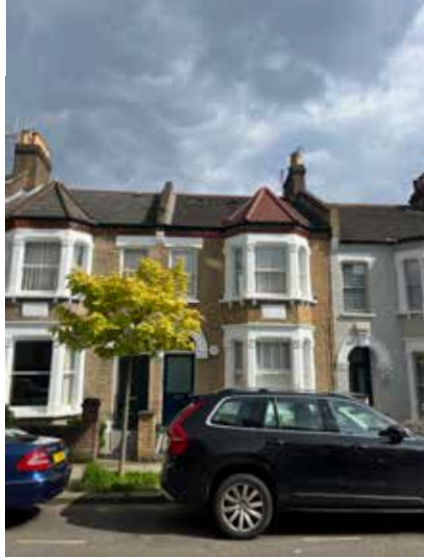
Existing front elevation. Picture taken: May 2024
