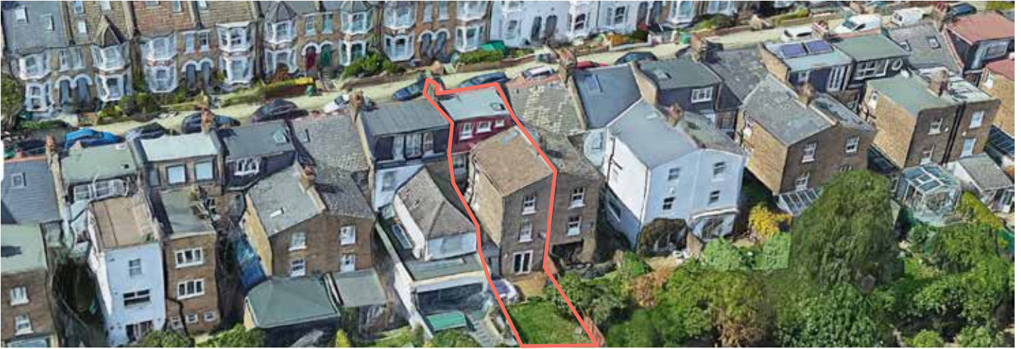
Aerial view of the property with the application site outlined.
