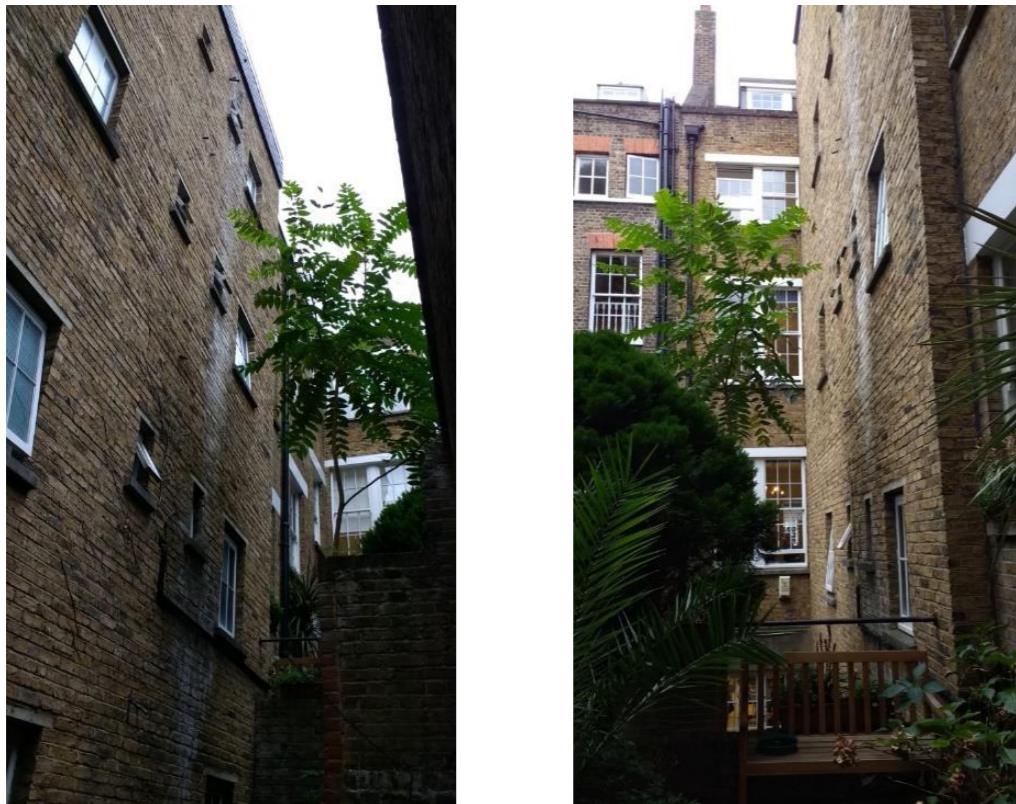
Figures 21 & 22: A view of the southern façade of the link block looking east and a similar view looking west towards the rear façade of no.9 John Street.
