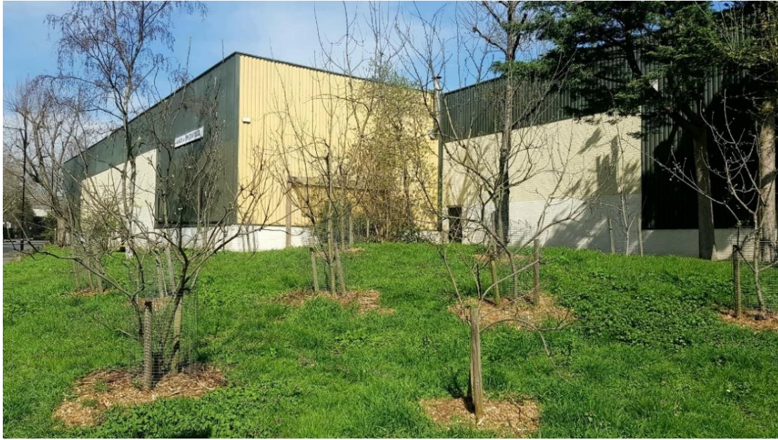
5. Planted 'orchard' at Camley Street/Cedar Way junction
