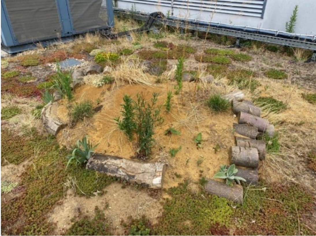
Fig. 4 green roof with sand mound in open mosaic habitat
