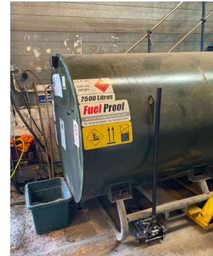
2500 litres above ground gas oil diesel tank within the Idverde unit, to the south of the shutter door.
