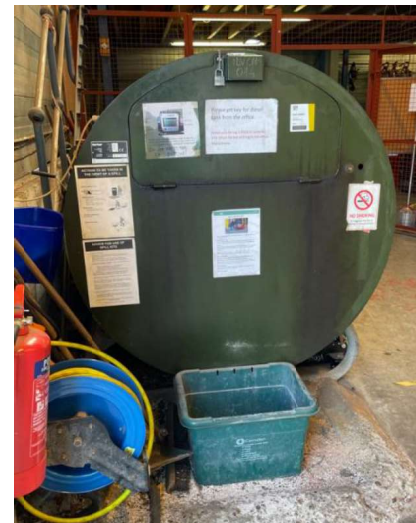
2500 litres above ground gas oil diesel tank within the Idverde unit, to the south of the shutter door.
