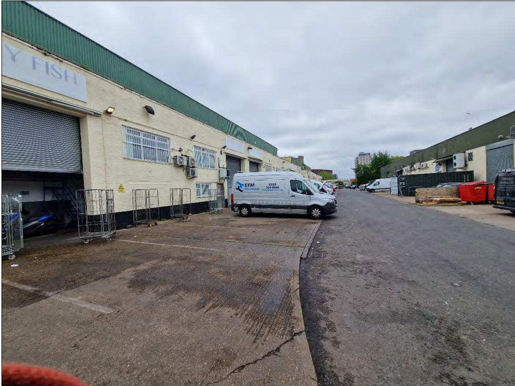
Plate 5) View from the northern end of Cedar Way, facing south
