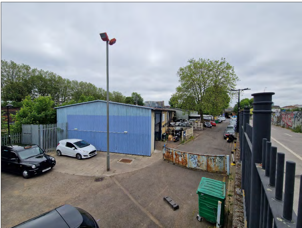
Plate 2) View from the southern section of Site A, facing south
