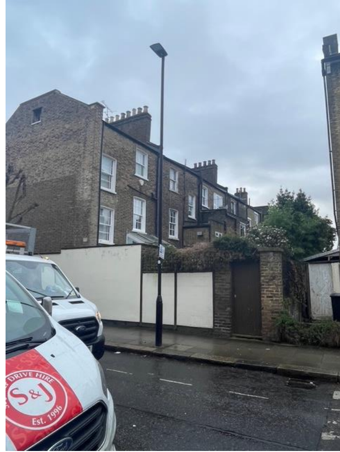
Figure 3. View of Side and rear elevation from Patshull Road
