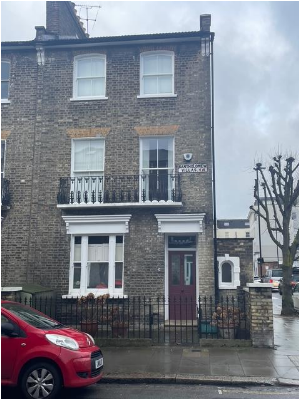
Figure 1. View of the front façade of n.42 Bartholomew Villas
