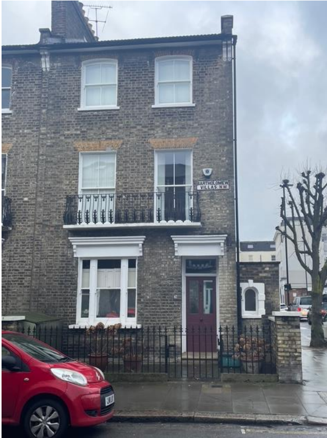
Image of N.42 Bartholomew Villas
