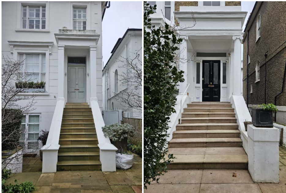
Existing Photos : York stone steps to neighbouring properties along Eton Villas and Steele's Road
