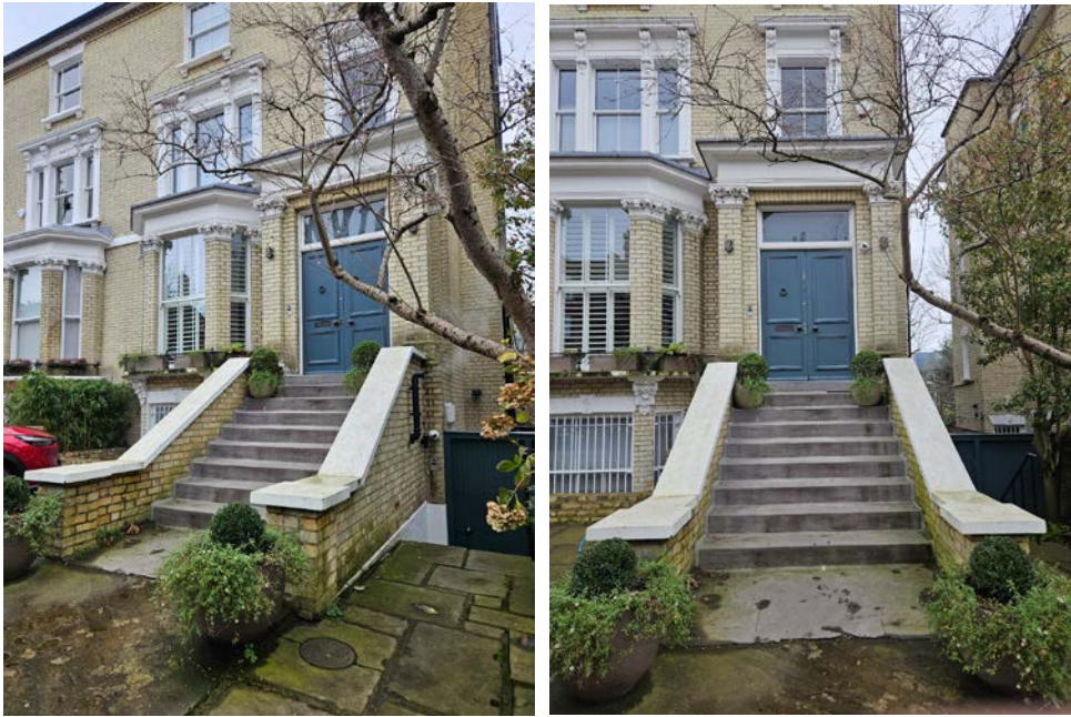
Existing Photos : Front Entrance
