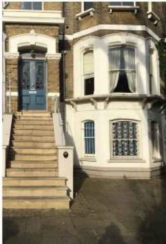
Ground and 1st floor (flat 1) at the front.
