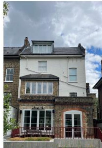
1st floor (flat 1), 2nd floor (flat 2), 3rd and 4th floors (flat 3) at the rear.
