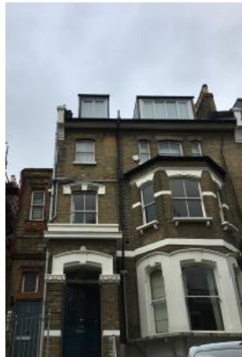
1st floor (flat 1), 2nd floor (flat 2), 3rd and 4th floors (flat 3) at the front.
