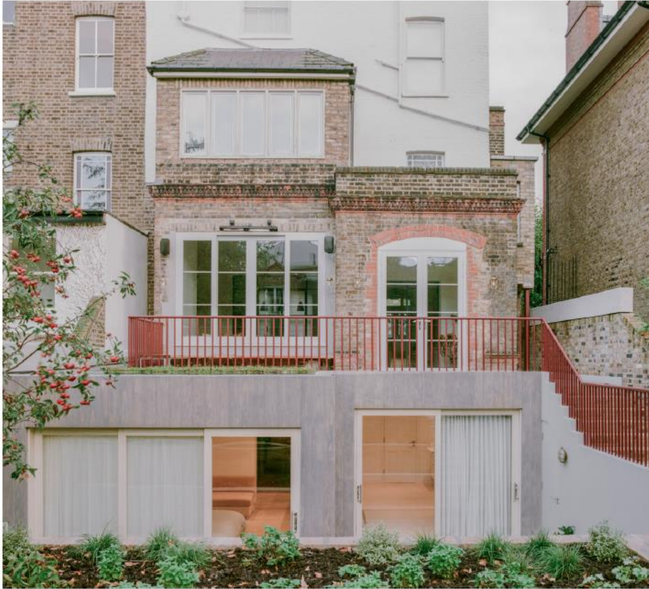
Ground and 1st floors (flat 1), and view of 2nd floor (flat 2) at the rear following 2020 extension and renovation of Flat 1.
