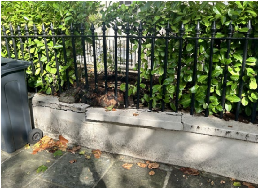
3. Existing drive (top), timber fence (middle) and boundary wall to drive area (bottom)
