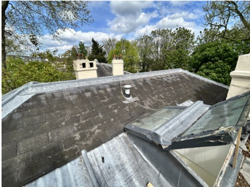
4. Existing valley roof of main building
