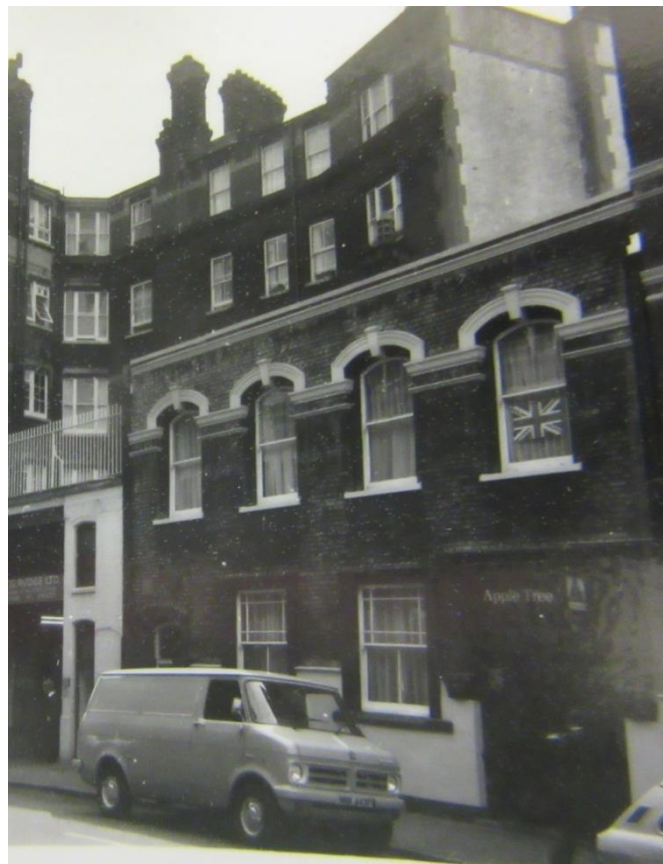
Figure 19: The Apple Tree (the 1925 extension, north elevation) in 1977.
