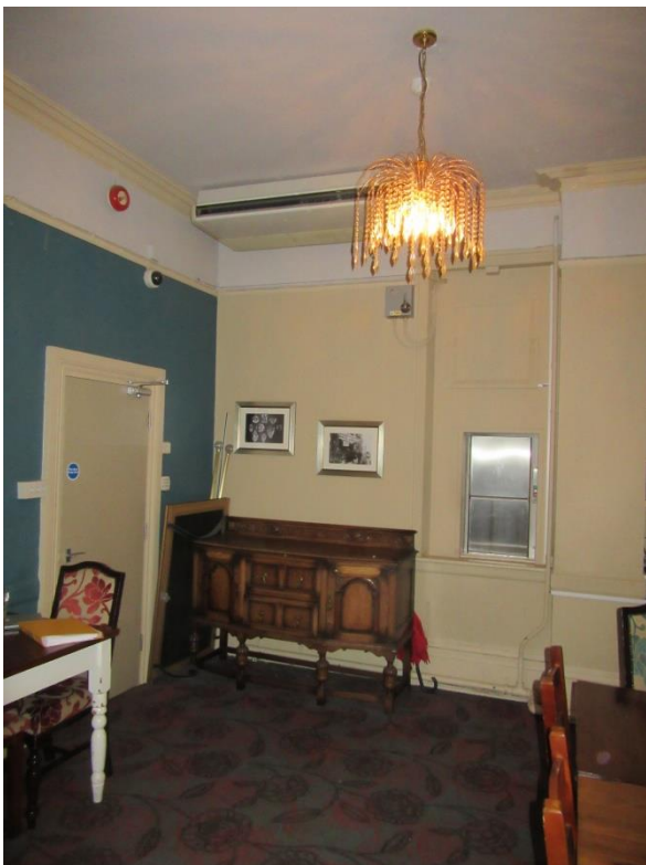
Figure 33: The rear part of the function room, formerly a separate room, showing modern door and dumb waiter within blocked window opening.
