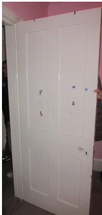
Figure 39: Altered 19 th century second-floor door.
