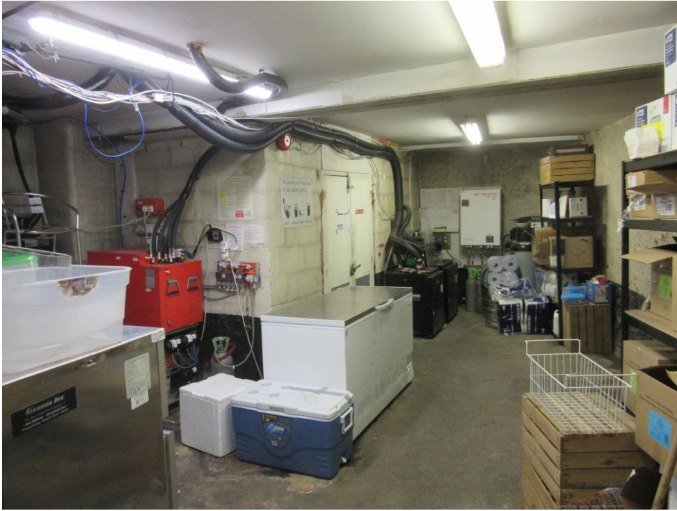
Figure 28: The original basement area beneath the 1870s public house, showing partitioned beer store with original brick pier (left) and barrel chute (adjacent to storage rack right).
