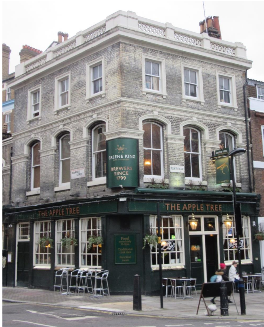
Figure 23: The principal north and west elevations of the 1870s building fronting Mount Pleasant and Warner Street.
