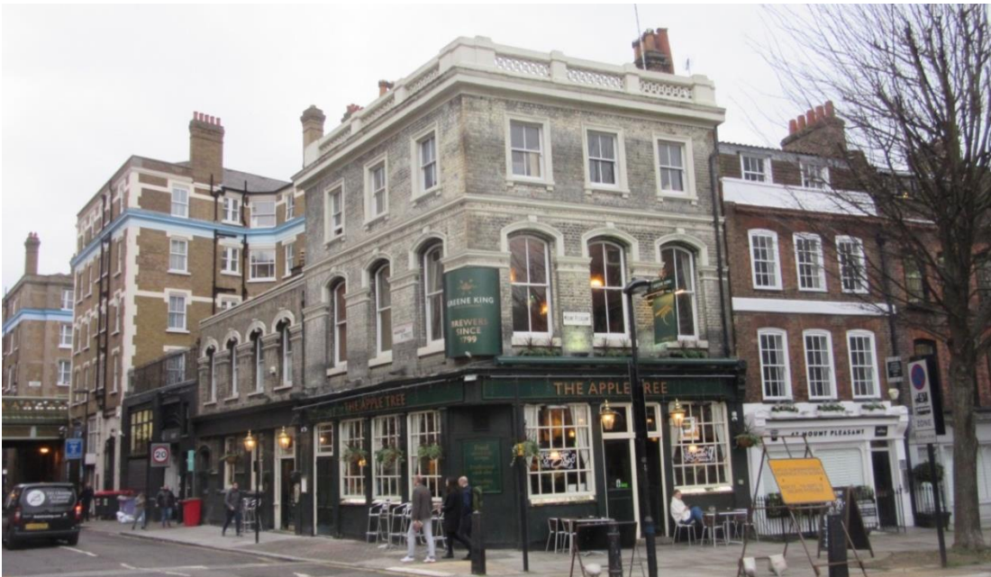
Figure 2: The streetscape context of the subject site, depicting the adjoining Grade II statutorily listed former townhouses on Mount Pleasant (right), the Grade II statutorily listed viaduct over Warner Street (left), and the 1890s residential blocks at Rosebery Square (left middle).
