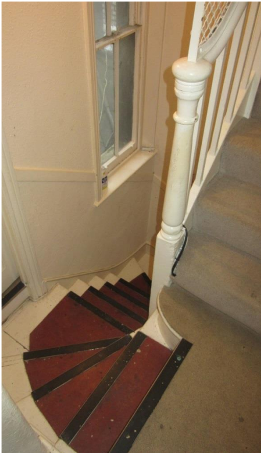
Figure 37: The first-floor “landing” (left) providing access to the different phases of the building and stairs to the second floor (right), illustrating the original staircase with moulded newel post.
