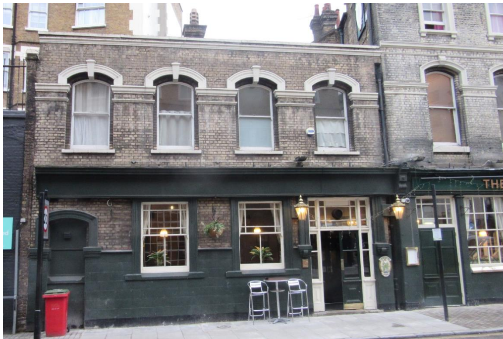
Figure 24: The Warner Street elevation of the 1925 extension which is largely intact with the exception of the covered faience and blocked doorway to the east bay.
