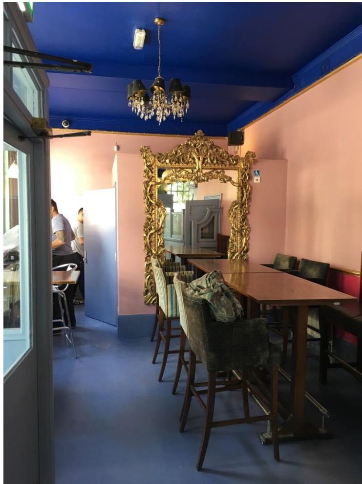
Figure 31: The 1925 extension looking east; there is little or no fabric of any historic interest in this area.
