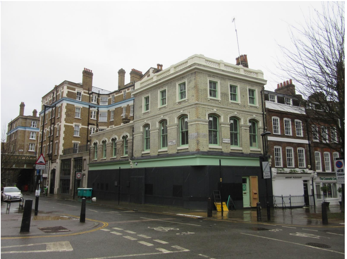
Figure 1: The external elevations fronting Mount Pleasant and Warner Street; all windows have been replaced as per the consent, although the ground floor remains boarded.
