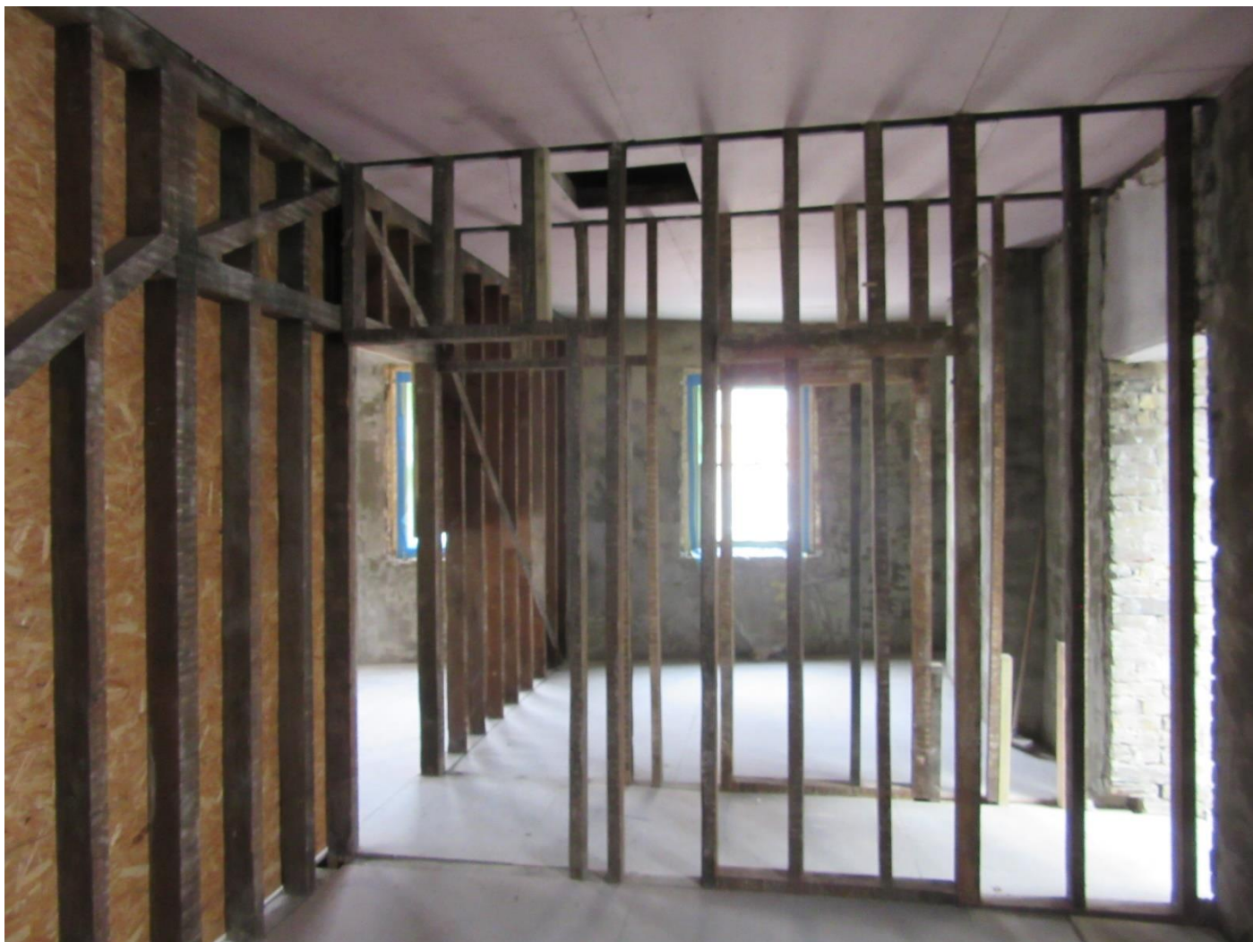
Figure 9: The rear part of the second floor with historic studwork.
