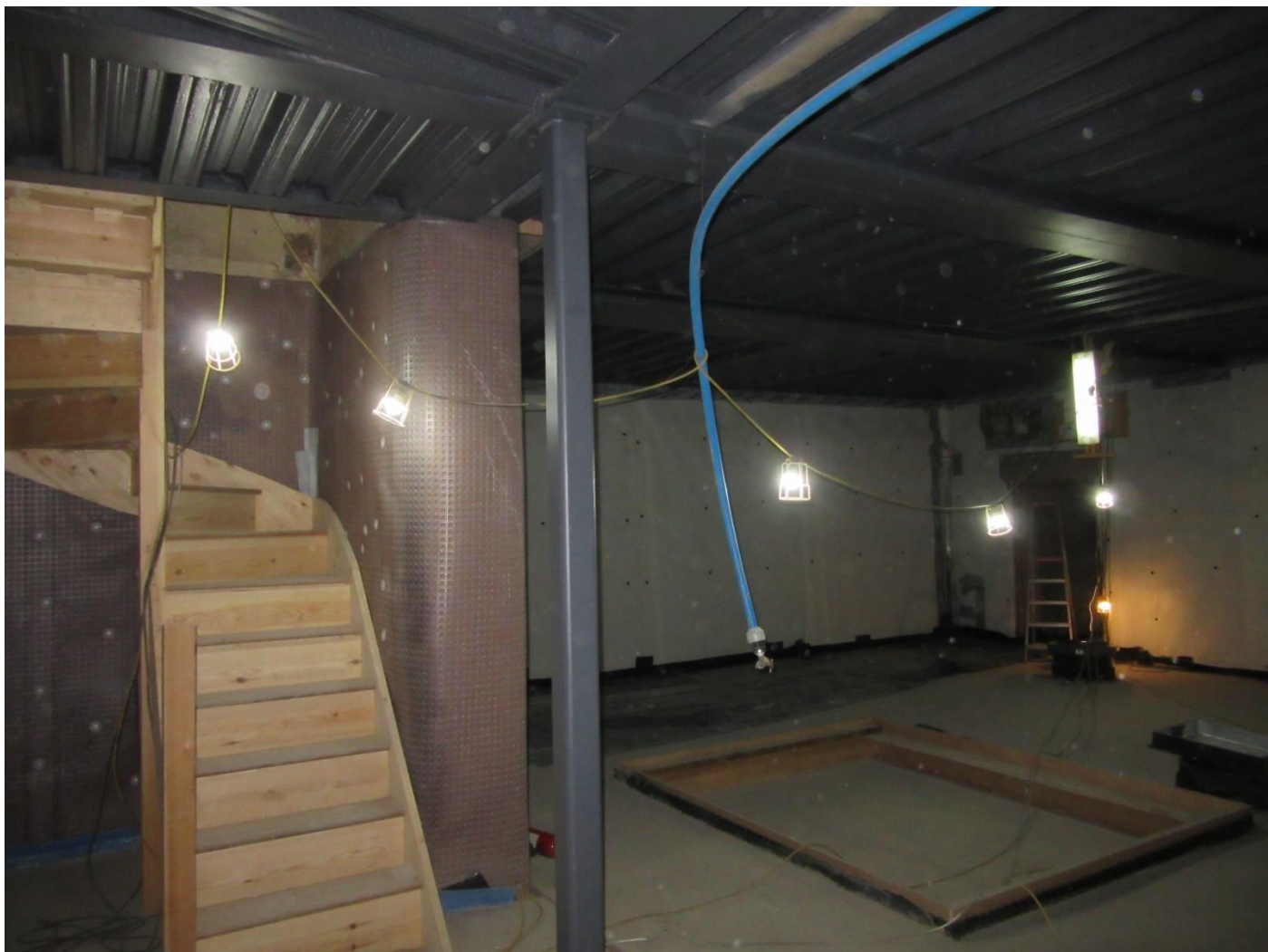
Figure 5: The basement with the consented rebuilt stair and reconstructed ceiling.
