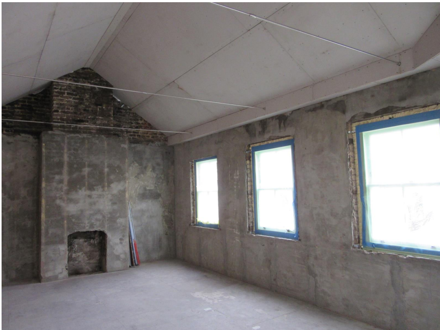
Figure 8: The second floor front room with incomplete finishes.
