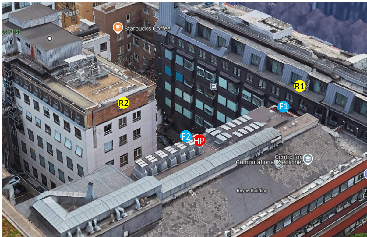
Figure 3.2 Aerial view of site with survey location (F1, F2 blue), nearest receptor façades (R1, R2, yellow), and proposed ASHP location (red)
