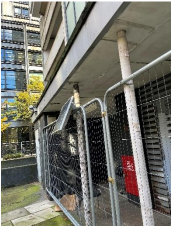
Photograph 3 Monitoring location A3
