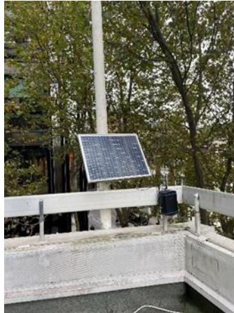
Photograph 2 Monitoring location A2
