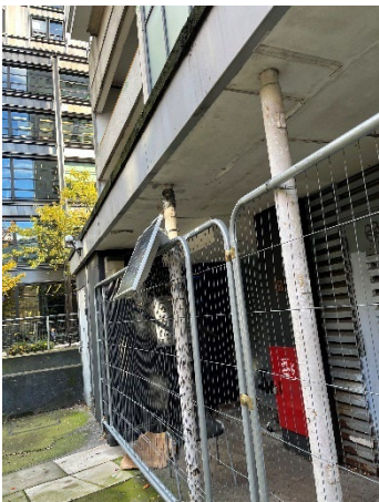
Photograph 3 Monitoring location A3
