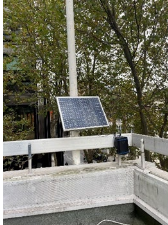
Photograph 2 Monitoring location A2
