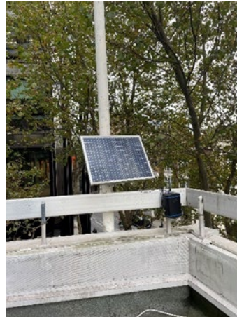
Photograph 2 Monitoring location A2
