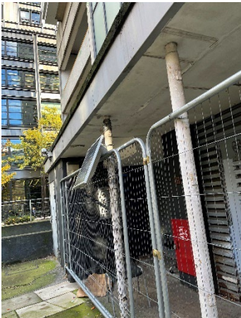
Photograph 3 Monitoring location A3
