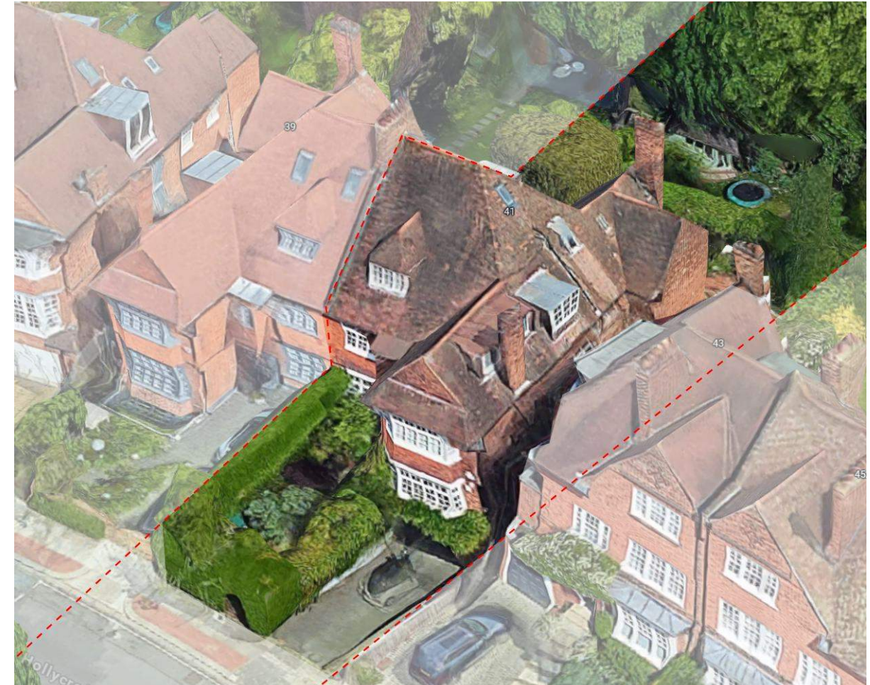
Aerial View of Site - Google
