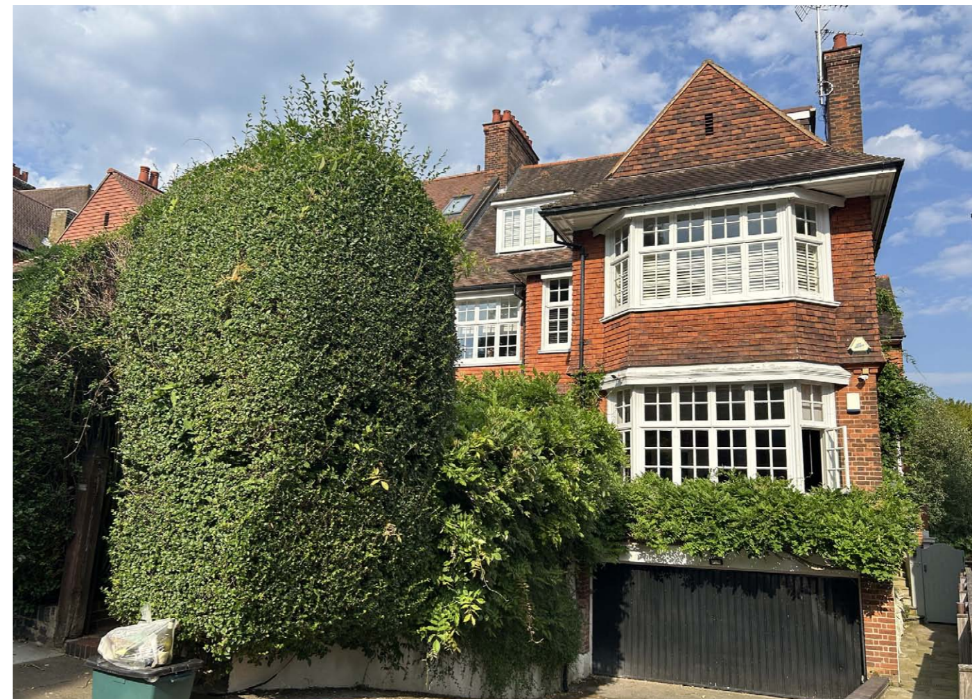
No. 41 Hollycroft Avenue seen from the street
