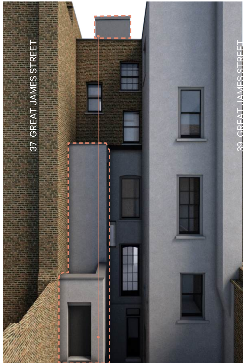
Fig. 4.1. Existing view of the rear elevation
