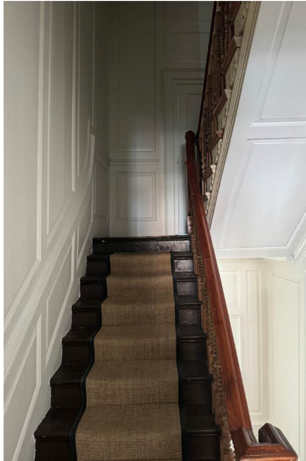
Fig. 2.12. First Floor stairs going to Second Floor
