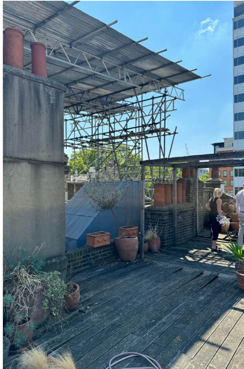
Fig. 2.21. Fourth Floor roof terrace looking South West
