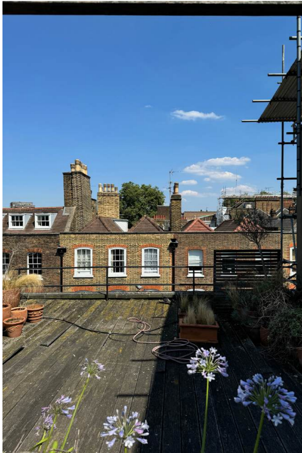
Fig. 2.20. Fourth Floor roof terrace looking East
