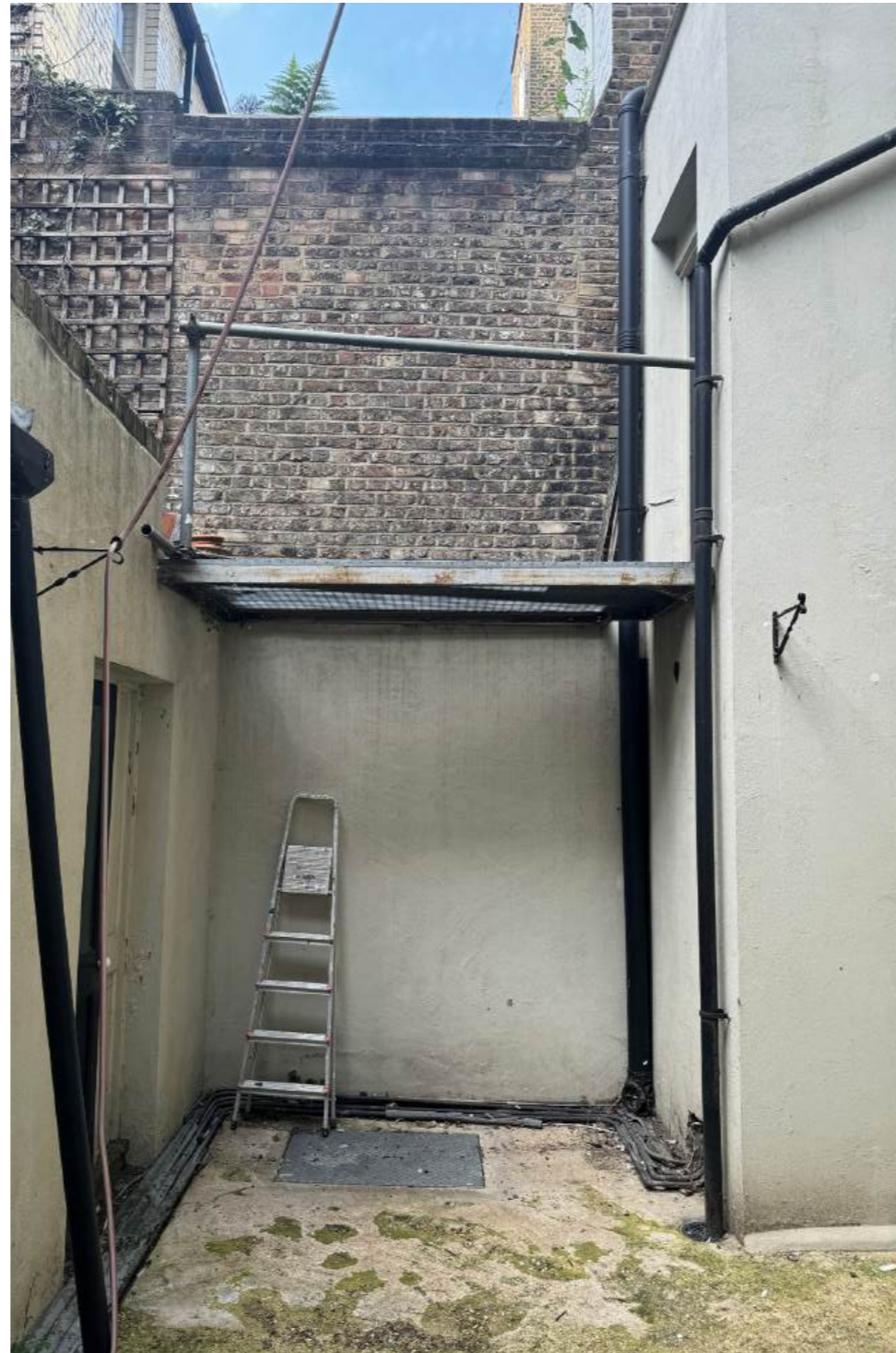
Fig. 2.9. Rear Garden boundary with 37 Great James Street looking North
