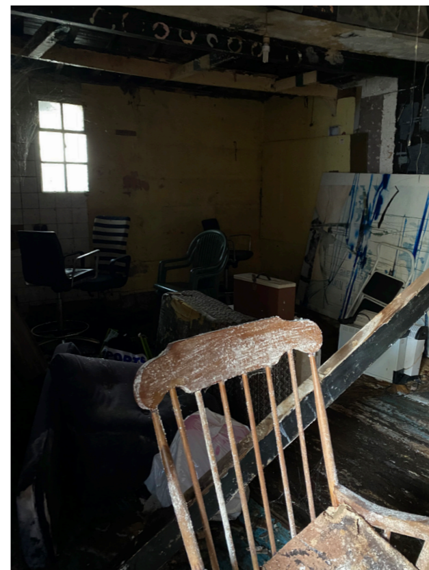
Existing interior of no.46 Inverness Street
